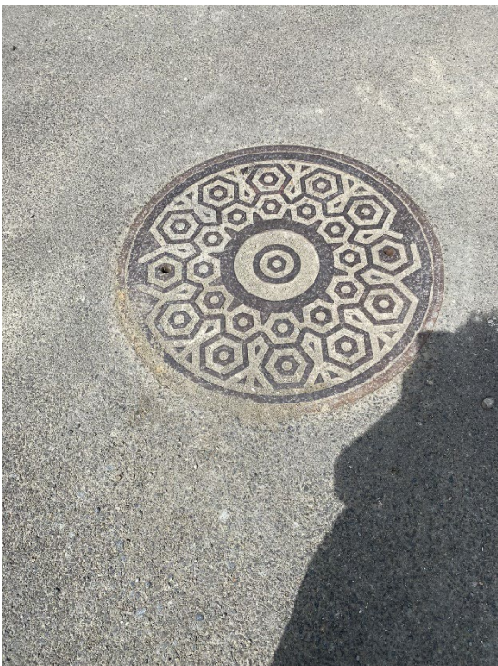
Photograph 7: Manhole, August 11, 2023, photo taken by Tetra Tech, Inc.
