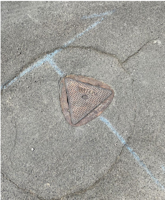
Photograph 6: Water access, August 11, 2023, photo taken by Tetra Tech, Inc.
