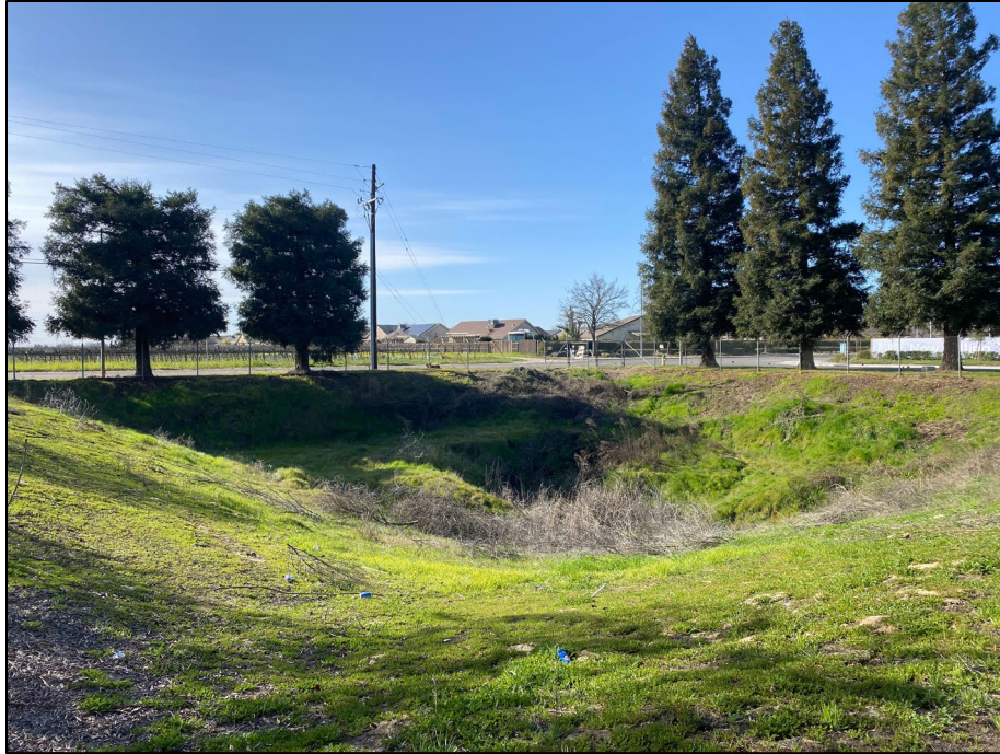
Figure 2a: Fowler Well Number 9 Project study area looking toward the intersection of E. South and Stanford Avenues. View toward the southwest.
