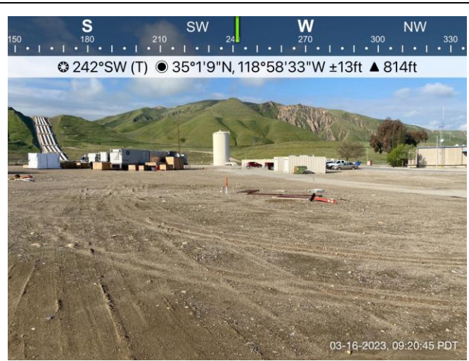
Photo 2. View of staging area from the north side.
