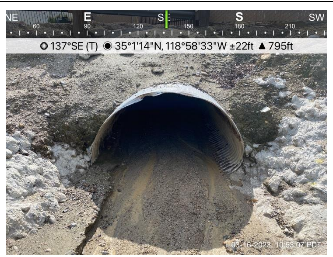
Photo 6. View of existing culvert.
