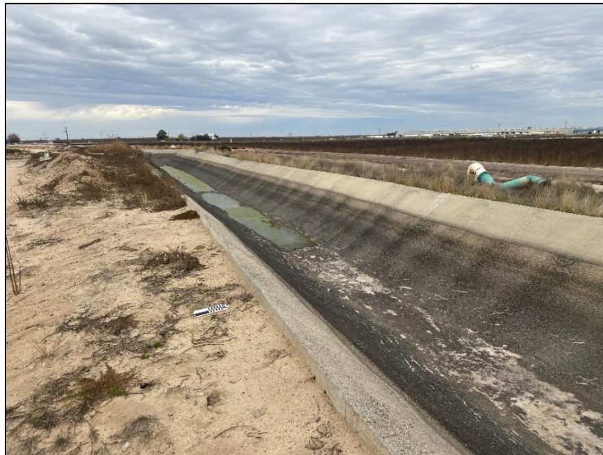
Figure 17. Overview of the Lateral Q bisecting the Project APE, looking west.
