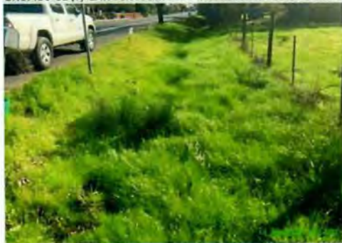
Photo 3 Looking South at shallow portion of roadside ditch that traverses the property along Old Redwood Hwy.
