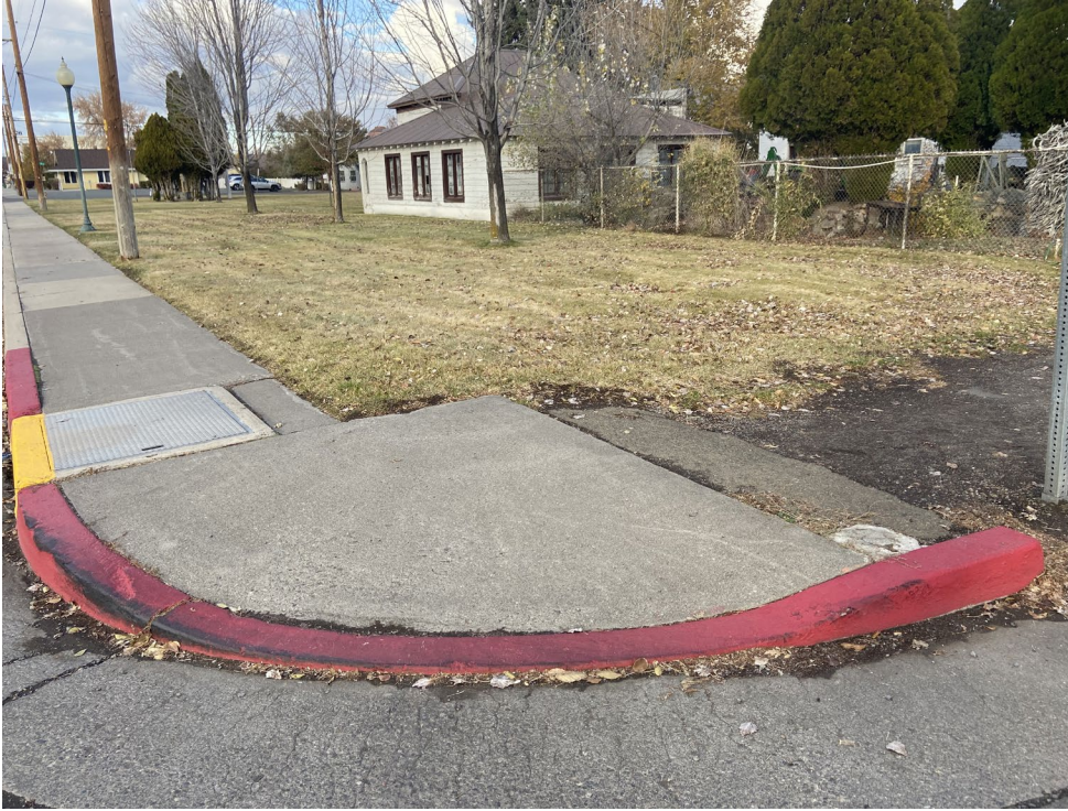
Photo 1. New right of way.
