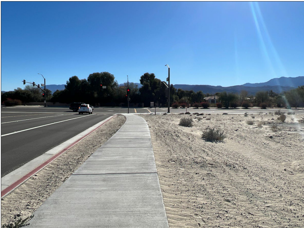
Photo 12. View of southeast corner of site (intersection of Ramon and Rattler Roads).
