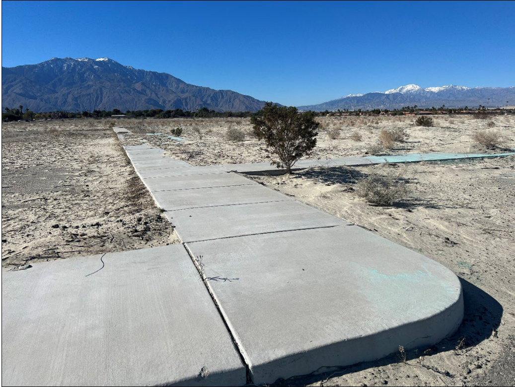
Photo 13. Remnants of a structure that was formerly present on the southeast corner of the site.
