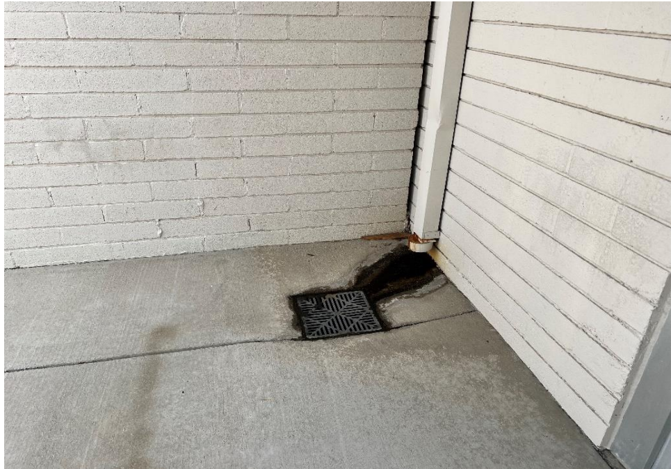
Photograph 11: View of gutter drain at the southern side of the building.
