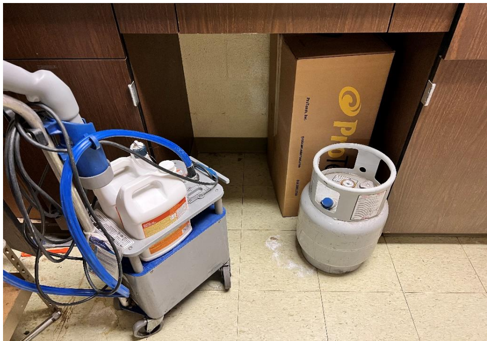
Photograph 8: View of approximately 5-gallon propane tank in the basement beneath the eastern portion of the property.
