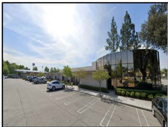
PHOTO 1: View of the northern portion of the project site along Upland Avenue.
