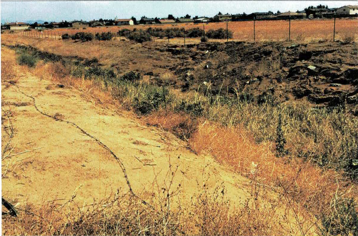
Photo #2: North-South storm control ditch.
