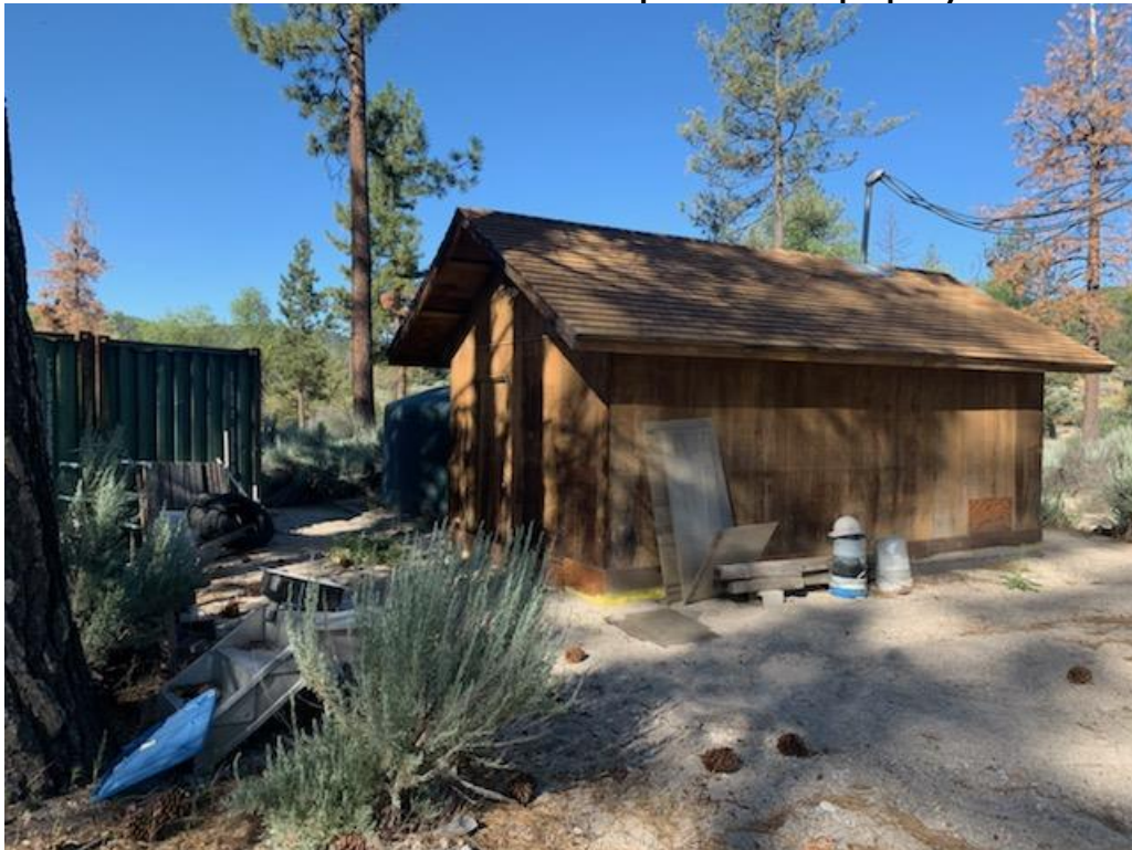
2. View of wood-frame structure on the northeast portion of the property.
