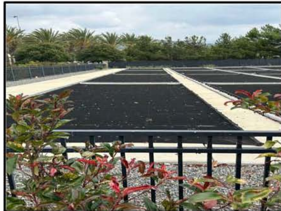
PHOTO 3: View looking east toward the existing solar array.
