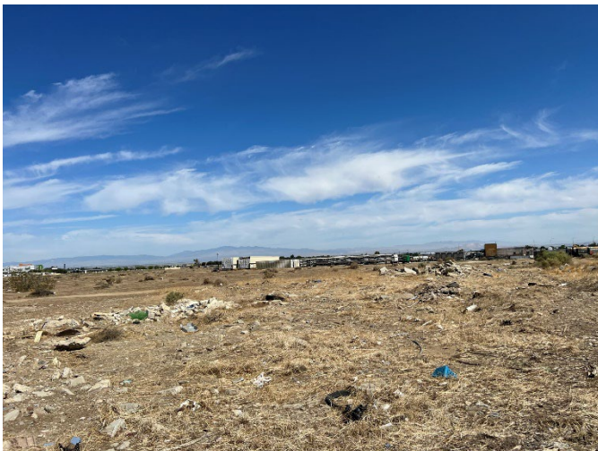
View of concrete piles in the northeast portion of the subject property
