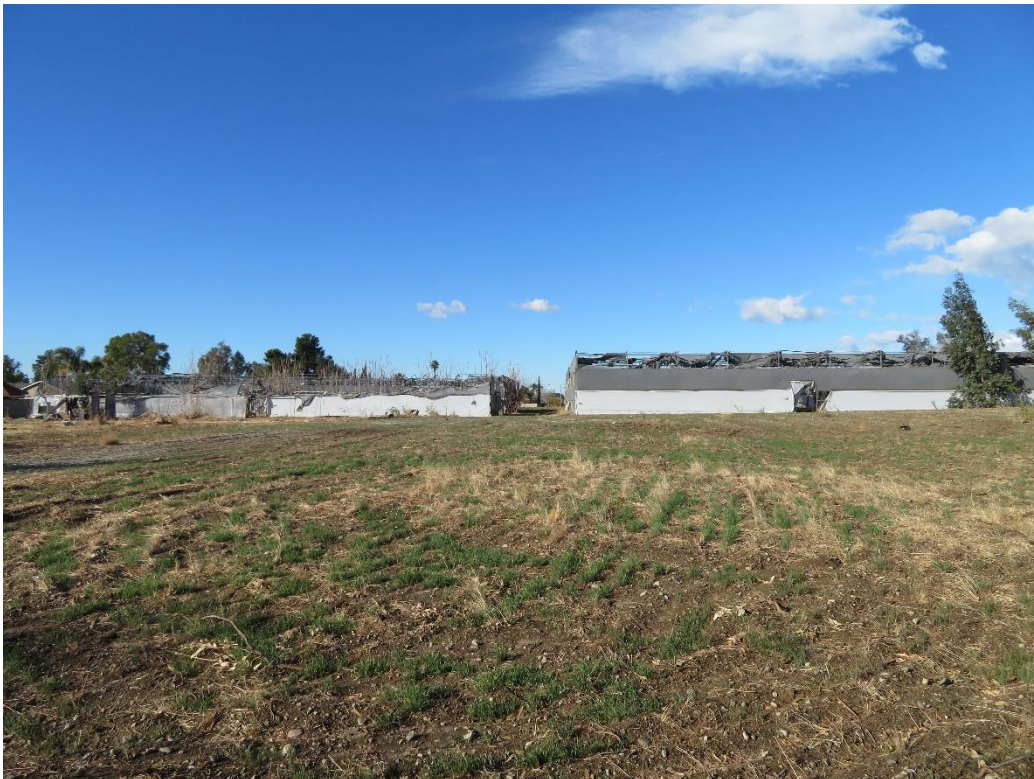
Photograph 6: Standing in the eastern portion of the project site, facing west. The remnant greenhouse structures can be seen in the distance.
