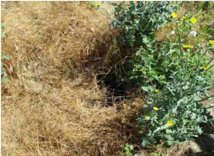
Photo #27: View of hole in the ground above the septic tank located behind (west of) the residence at 9092 Catawba Avenue
