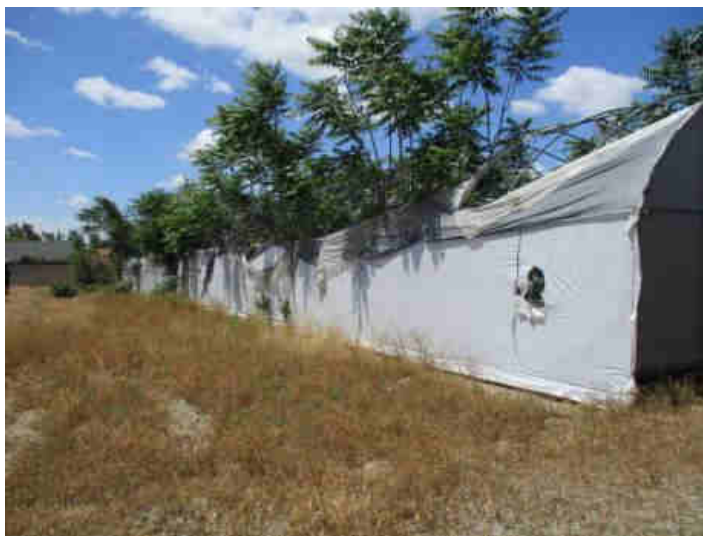
Photo #21: View of one of four abandoned greenhouses located onsite, looking south
