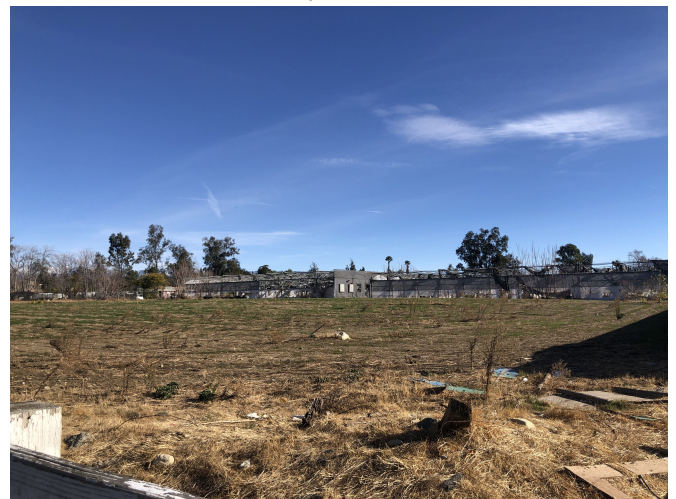
Eastern view of the existing abandoned greenhouses on the project site.
