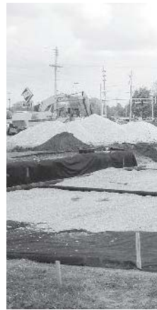
Place clean, crushed stone 9" (230 mm) min. thick. Compact to achieve 95% relative density.
