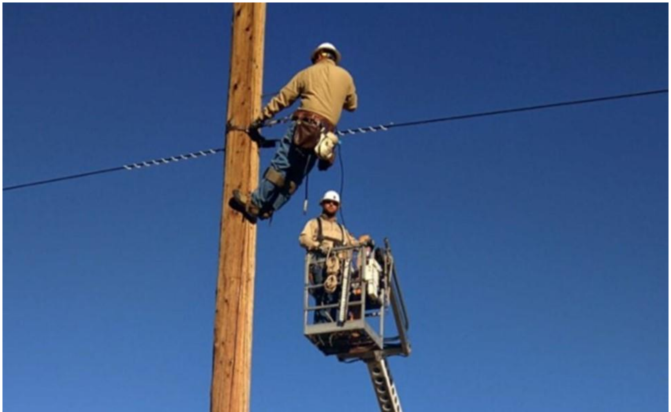
Figure 3. Segment 1 ADSS Installation on Distribution Pole
