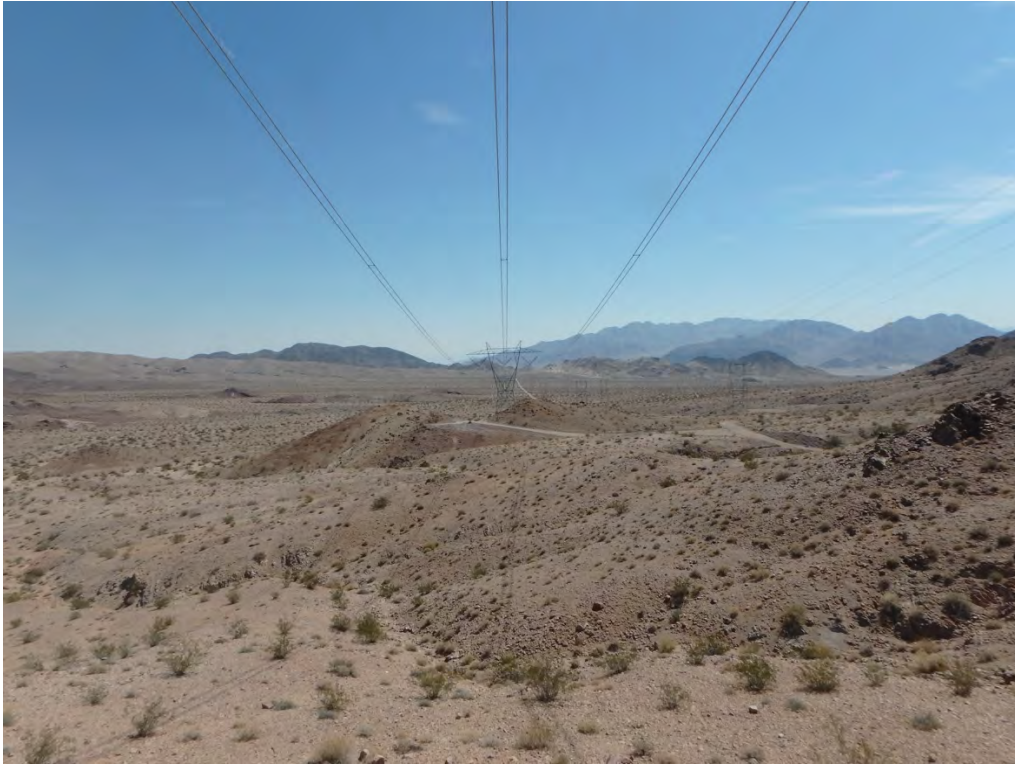
Figure 3. View of Qa valley with hills in foreground and background composed of mixed igneous and metamorphic rock. View to north.
