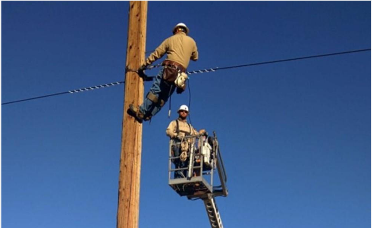
Figure 3. Segment 1 ADSS Installation on Distribution Pole
