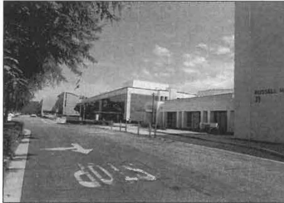
View 8. From east side of the project site, looking southeast towards the Planetarium (Building M), the Administration Building (Building S), and the Cesar Chavez Building (Building A) that are to the east of the project site.
