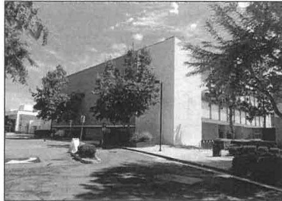
View 2. From parking lot 1, looking southwest towards Russell Hall (Building R) on the project site.
