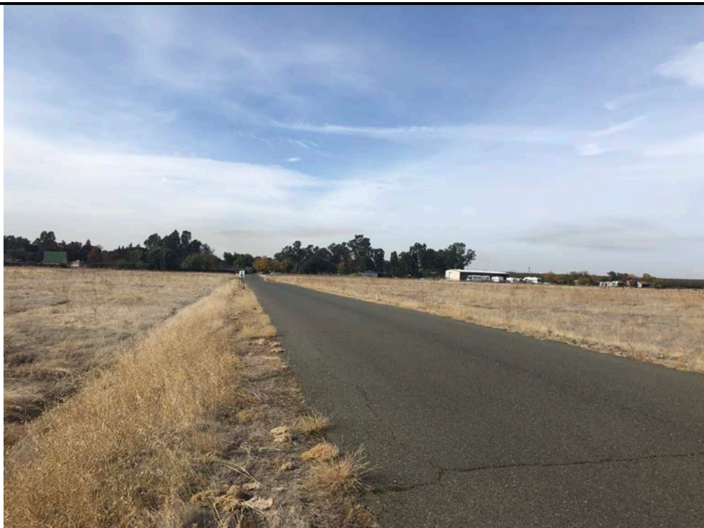
10. Facing west, photo shows the Airport Access Road that delineates the northern Property boundary. Ephemeral drainage ED1 can be seen on the left-hand side of the access road.
