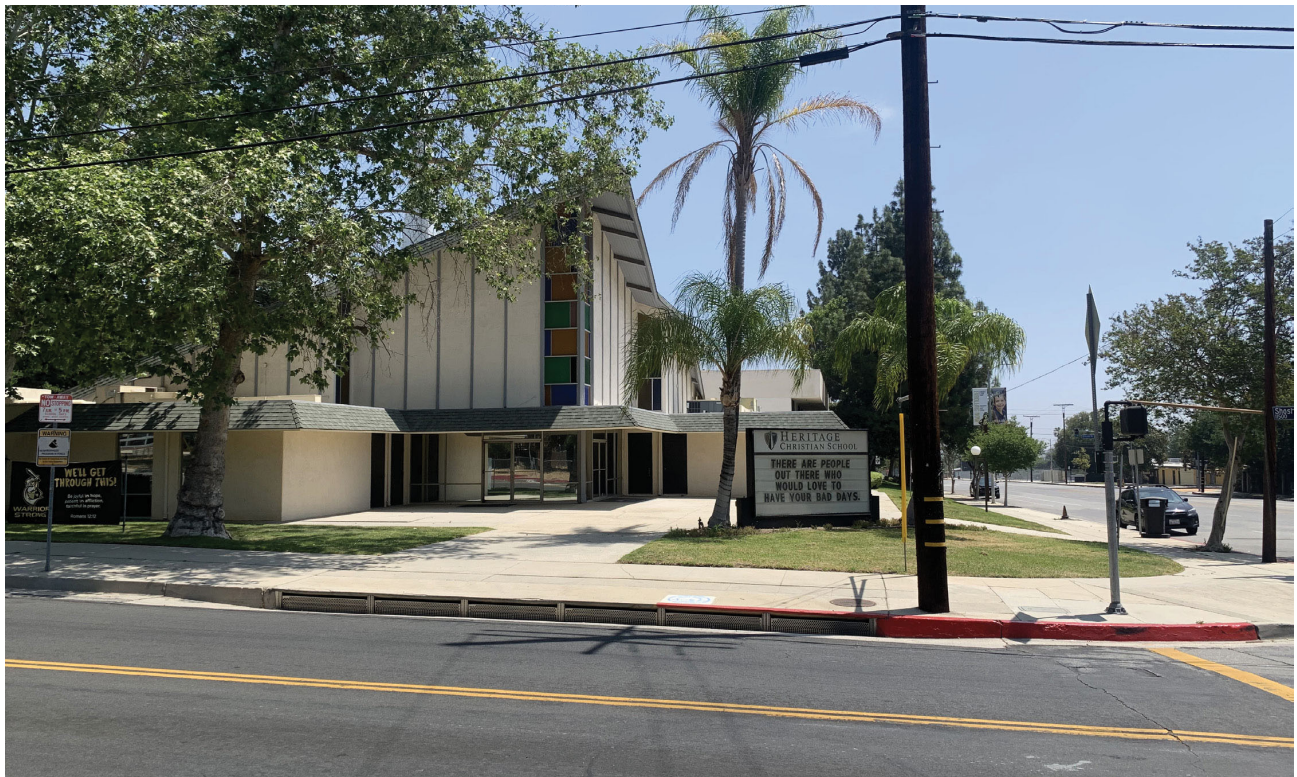
6. View looking east from Shoshone Avenue of the Heritage Christian School.
