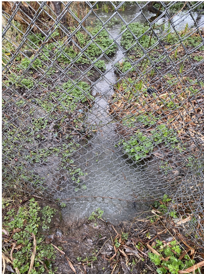
Northern discharge sampling location, D#2. Discharge received from subsurface corrugated pipe receiving runoff from concrete lined ditch and adjacent areas.
