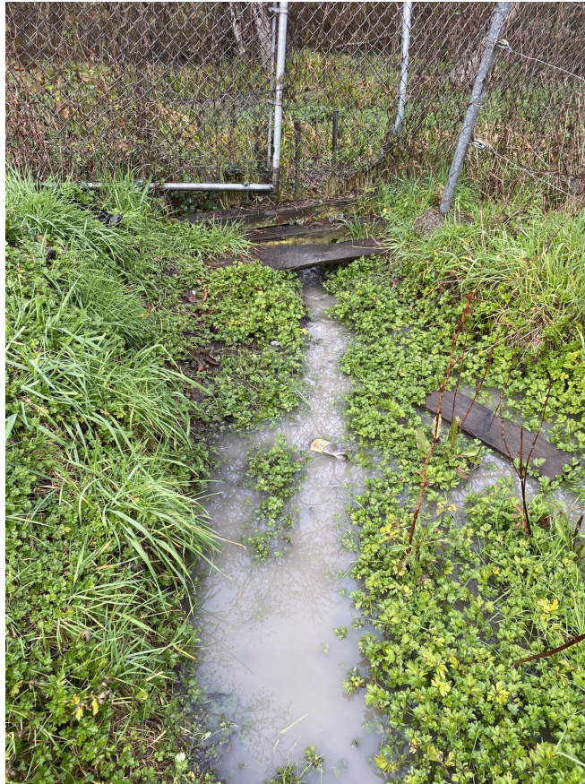
Southern discharge sampling location, D#1. Discharge received from vegetated swale receiving runoff from concrete lined ditch and adjacent areas.
