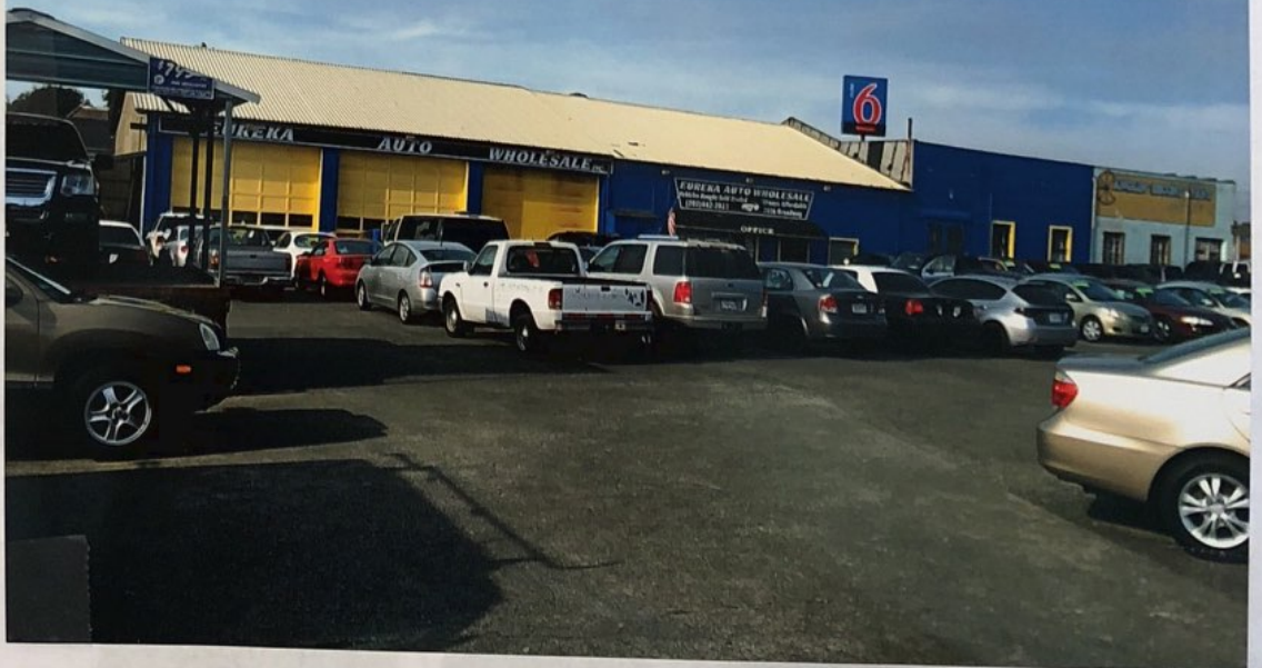
SOUTH WALL (ENDING JUST BELOW MOTEL 6 SIGN)
