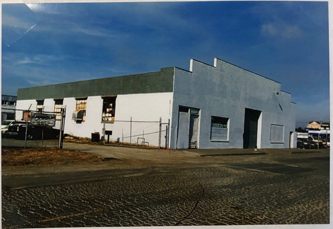
FACADE & WEST WALL
