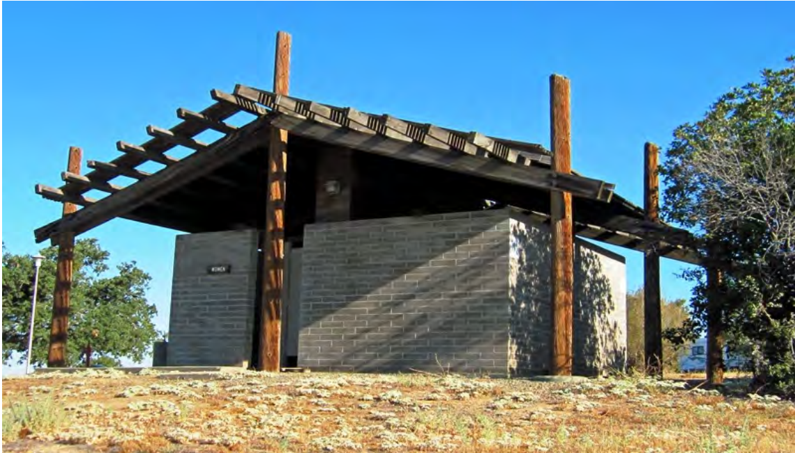
Blue Oaks Recreation Area Comfort Station south and east façades, View northwest, Photo taken 07/13/12
