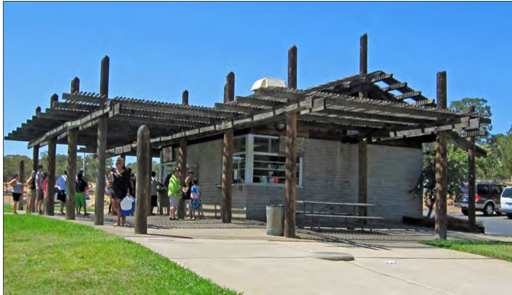
Fleming Meadows Recreation Area Snack Bar, south primary façade and east façade, View northwest, Photo taken 07/13/12
