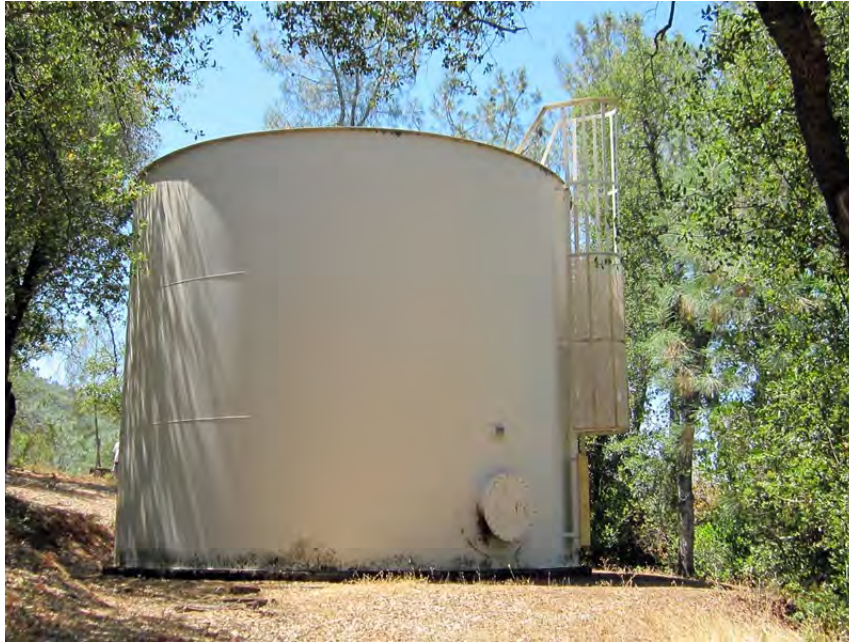
Moccasin Point water tank, View west, Photo taken 07/13/12
