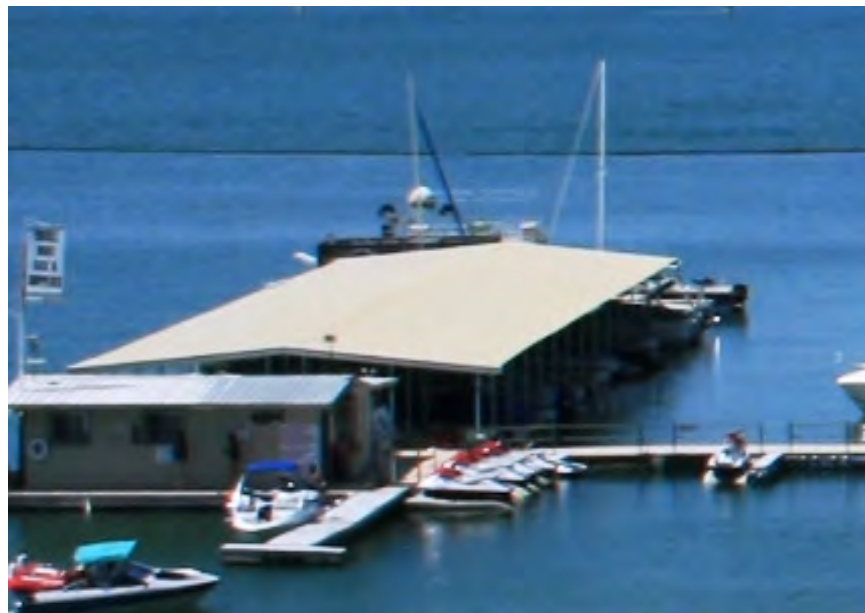
Fleming Meadows Recreation Area Marina, West Boat Shed, south primary façade and east façade, Photo taken 07/15/12
