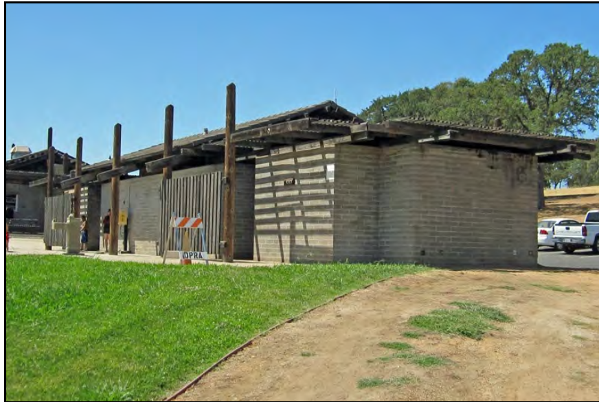
Fleming Meadows Recreation Area Dressing Rooms, east and west façades, View northwest, Photo taken 07/13/12
