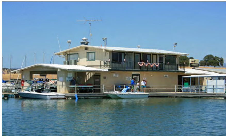
Fleming Meadows Recreation Area Marina Forever Resorts office and Marina Café south primary façade and west façade, View northwest, Photo taken 07/15/12
