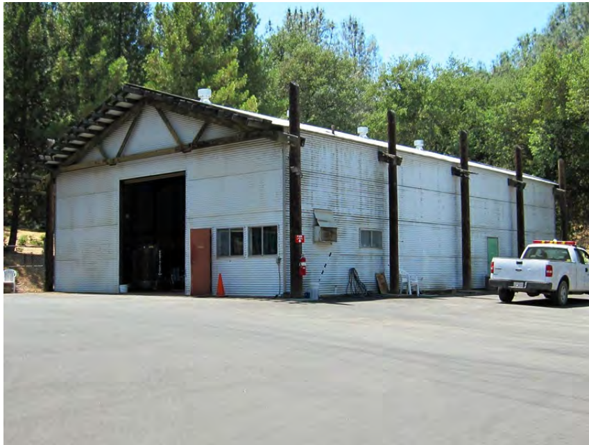
Moccasin Point Recreation Area warehouse, east primary façade and north façade, View west, Photo taken 07/13/12
