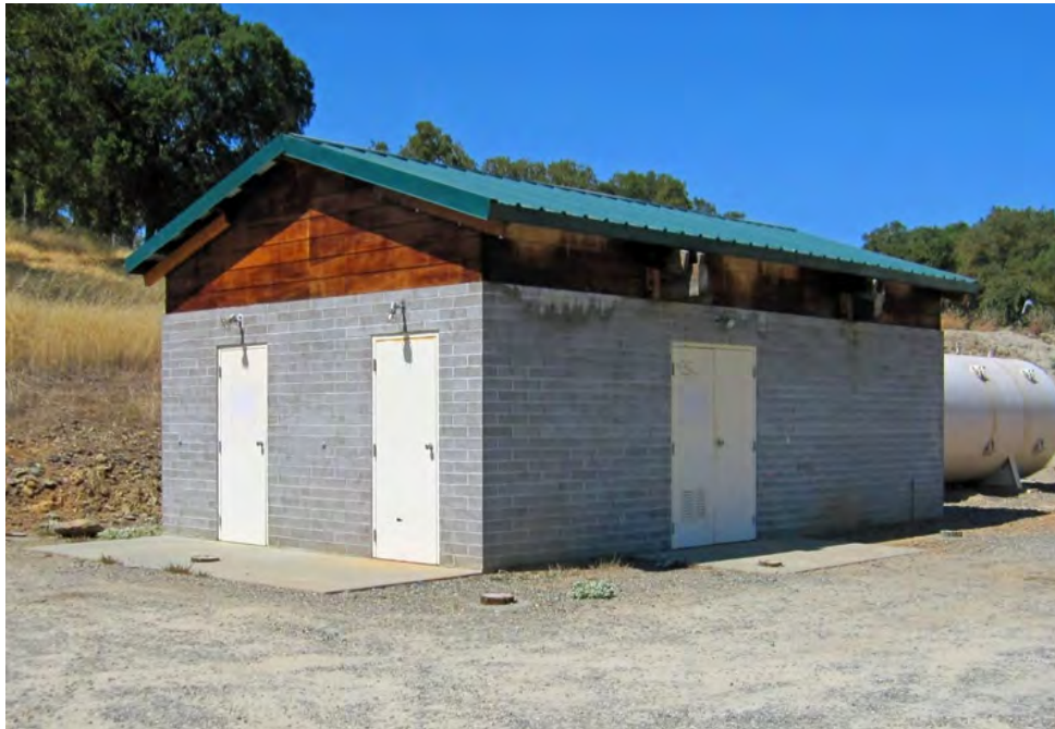
Fleming Meadows Recreation Area Water Treatment Building, west primary façade and south façade, View northeast, Photo taken 07/12.
