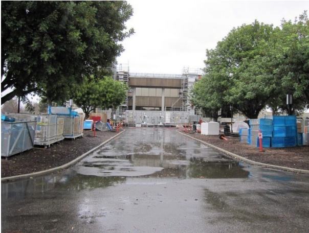
Photograph 1. View of the Site looking east toward Building SC1.
