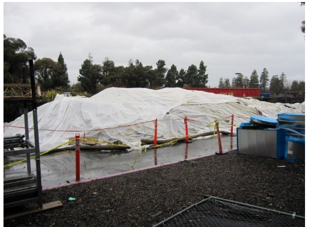
Photograph 4. On-Site stockpiled soil.
