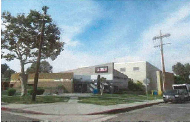
Photo 1: View of the front of the Watts Empowerment Center
