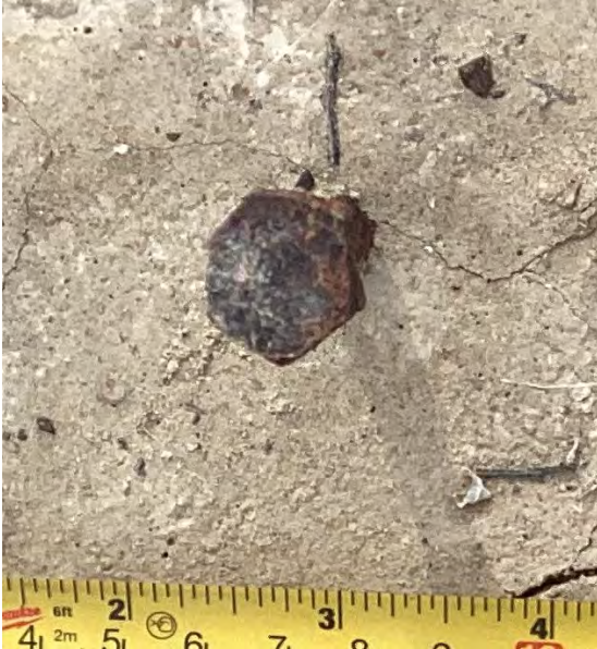
Wrought iron cut bolt top view (Photo #0368)
