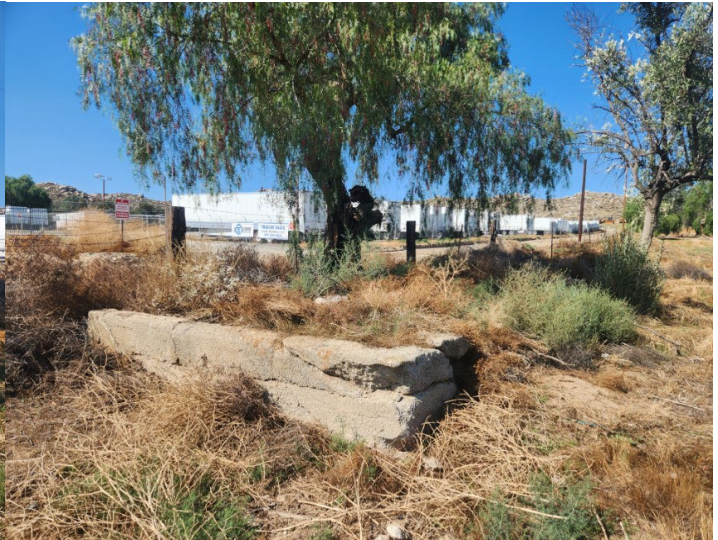
View southwest of northeast corner of foundation footing.
