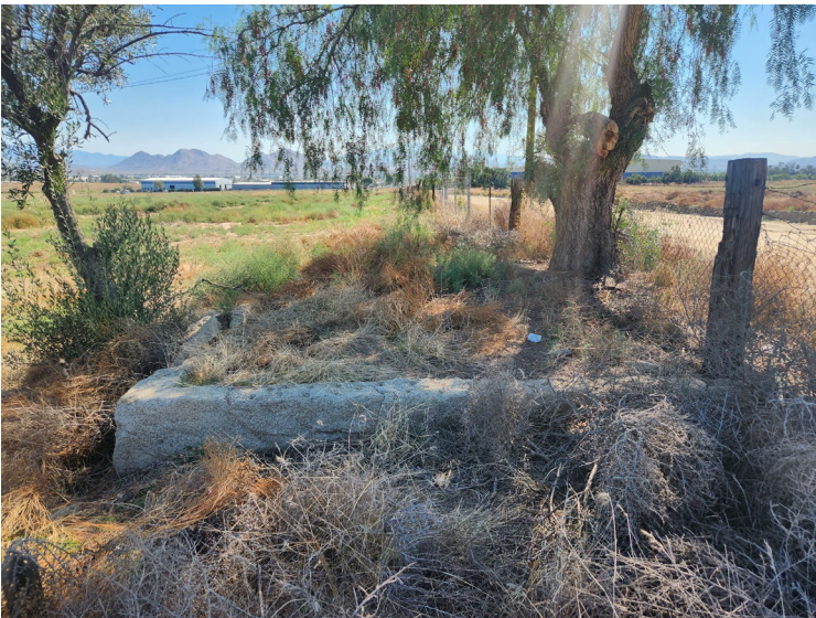
View east of west facing wall of foundation footing.
