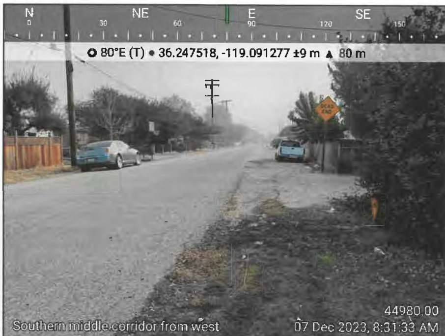
Figure 5. LSID Project study area corridor overview, looking east.
