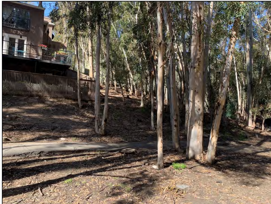
Photograph 4: Asphalt and sediments along the Glenwood Tributary. View to north.
