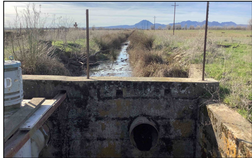
Photo 4. Outlet and distribution box for the ditch within the Study Area. Photo taken February 23, 2021, facing south.
