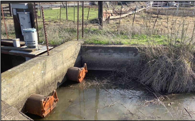
Photo 3. Outlet and distribution box for the ditch within the Study Area. Photo taken February 23, 2021, facing east-northeast.
