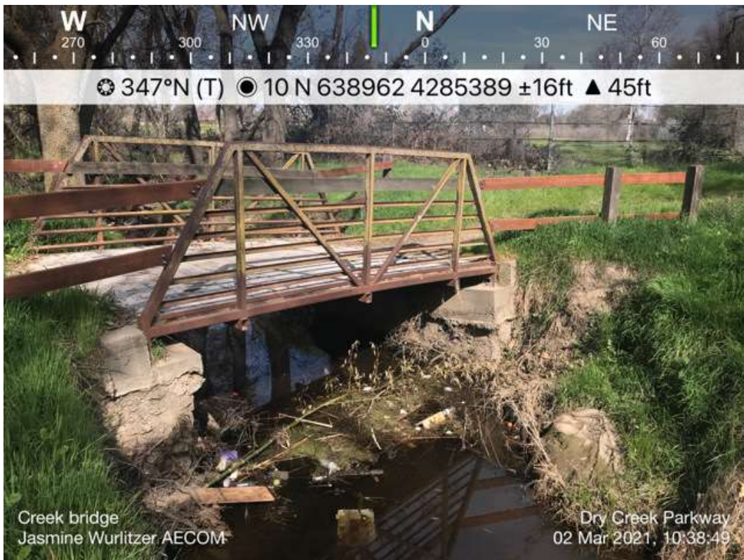
Photo 1. Aquatic Feature PR1 – Sierra/Goat Creek, existing bridge crossing.
