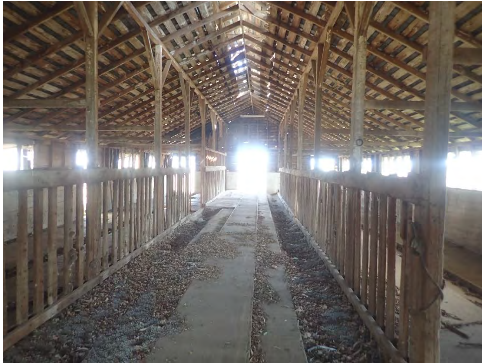
Photograph 5. Old livestock barn structure
