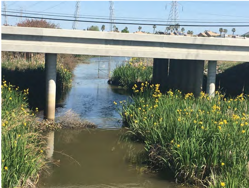
Photograph 11. Photograph 9. Bridge over Kellogg Creek at Hwy 4 (outside project site boundaries)
