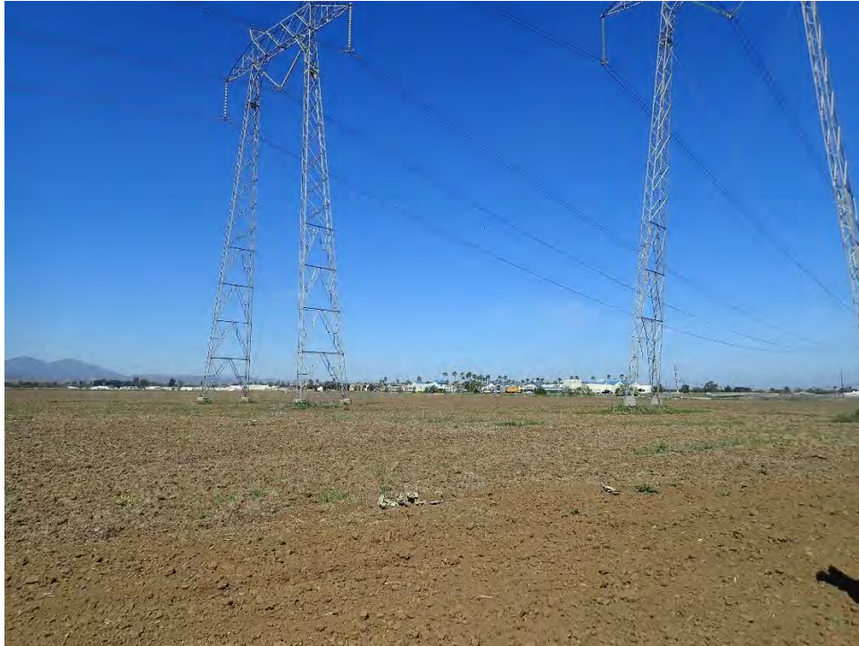
Photograph 7. Transmission towers in eastern portion of the site.
