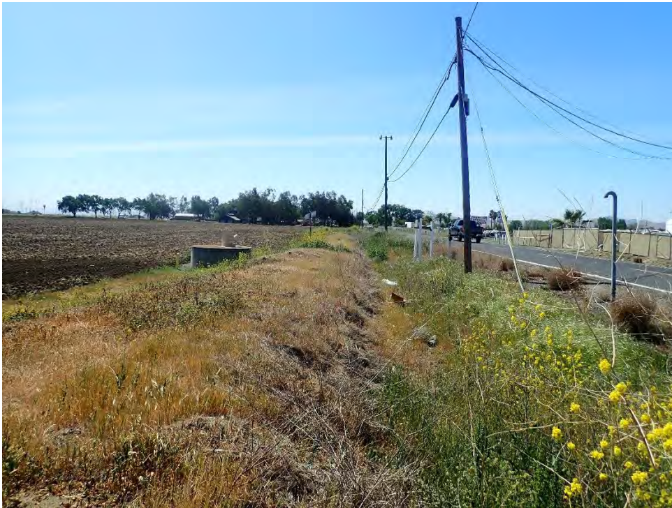
Photograph 8. Roadside ditch along Bixler Road (outside project site boundaries)
