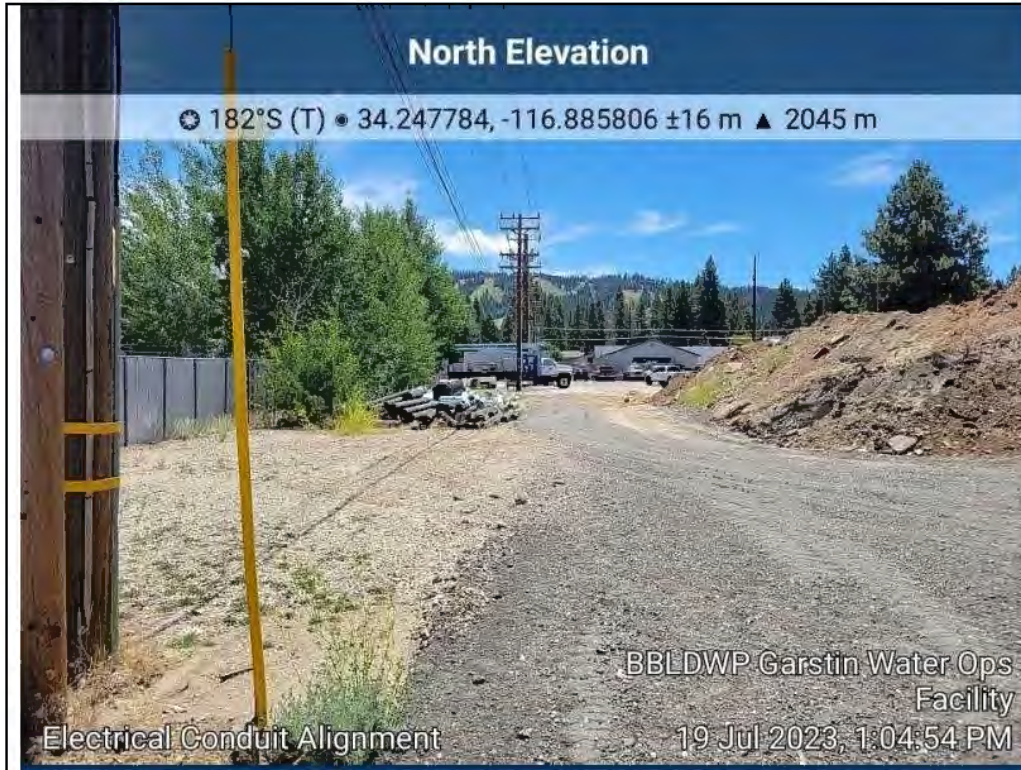
Photo 3. Proposed electric conduit alignment within existing disturbed BBLDWP property south of Fox Farm Road.
