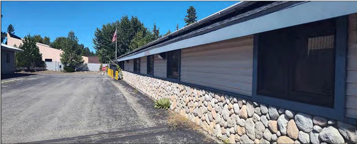
Rear (south side) of the operations building.
