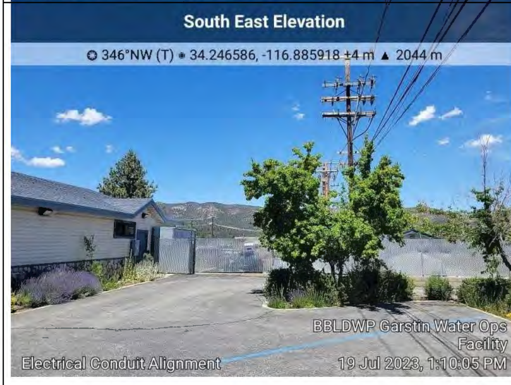
Photo 2. Southern end of proposed electric conduit alignment.
