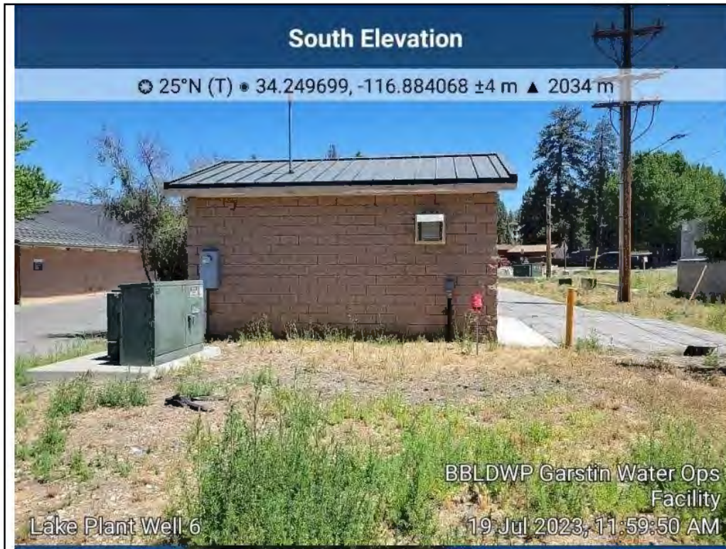
Photo 9. Existing Lake Plant Well No. 6.
