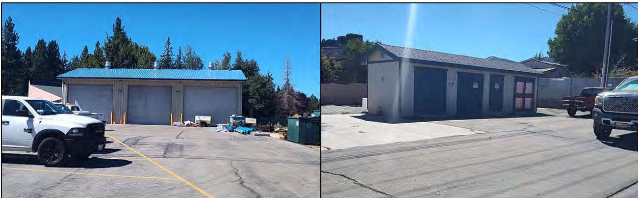
Maintenance garage, view to southwest (left); Powerhouse, view to southeast.
