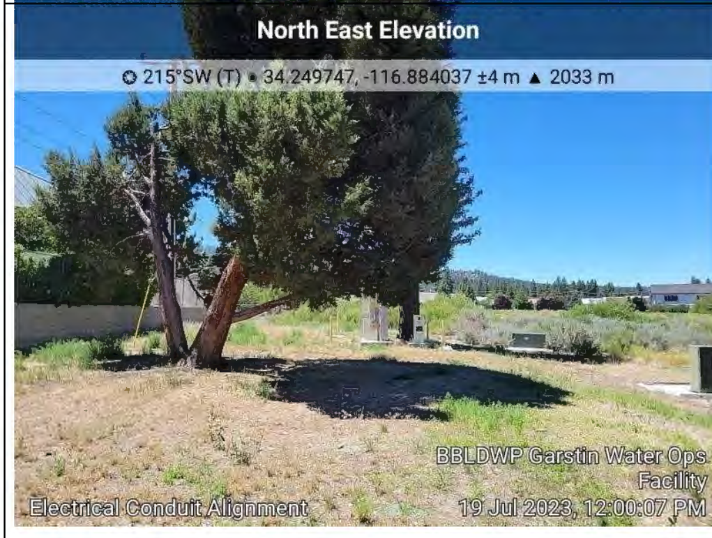
Photo 10. Proposed electric conduit alignment to existing Lake Plant Well No. 6, looking southwest from Lake Plant Well No. 6.
