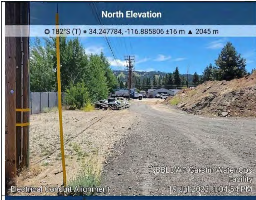
Photo 3. Proposed electric conduit alignment within existing disturbed BBLDWP property south of Fox Farm Road.
