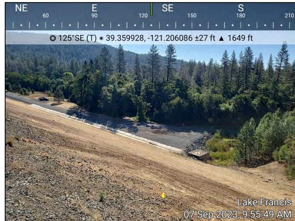
Photo Point 1. View of dam and access road at toe of dam. The low level outlet structure can be seen on the right side of the photo.
