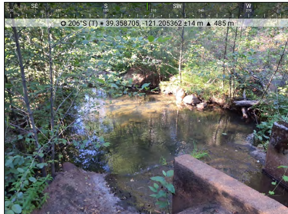
Photo Point 7. View of flume on Dobbins Creek.
