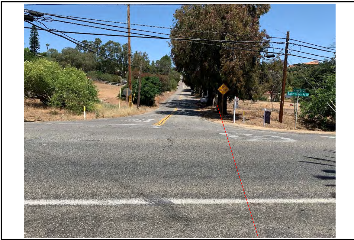
Photo Point 5. Photo taken at the intersection of Gopher Canyon Rd and Fairview Dr. Red line represents the approximate location of the alignment. Culverts are under the road at this location along with a non-wetland water (see Photo 7). Photo date: 05/05/22. Direction: north. Lat/Long: 33.2495, -117.22188
