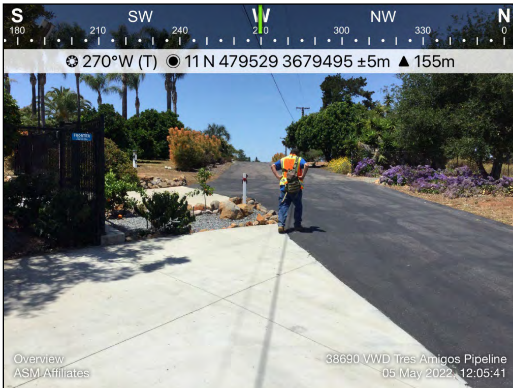
Figure 5. Overview of project alignment on Fairview Road showing residential paved roads.
