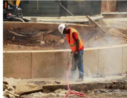
A worker breaks up concrete creating a cloud of silica dust.
