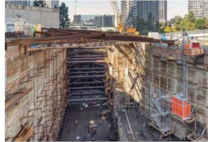
Excavation and shoring plans must be reviewed by Metro to ensure structural compatibility with Metro infrastructure and safety during adjacent development construction.
