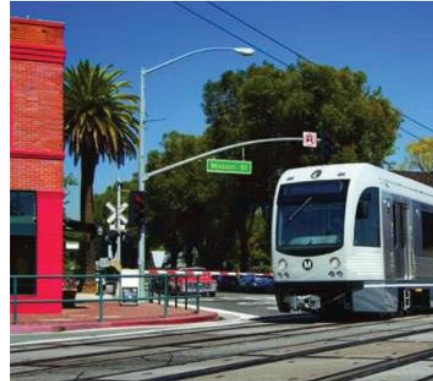
Gates and pedestrian arms are common types of safety elements for pedestrians at rail crossings.
