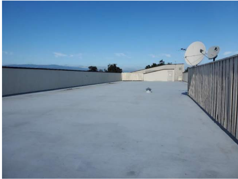
Photograph 33 – 5201 Patrick Henry Drive building roof
