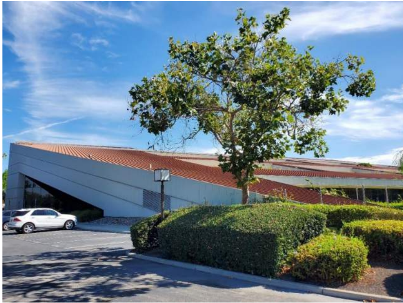
Photograph 3 – Southwestern side of the building, facing northeast from Patrick Henry Drive.
