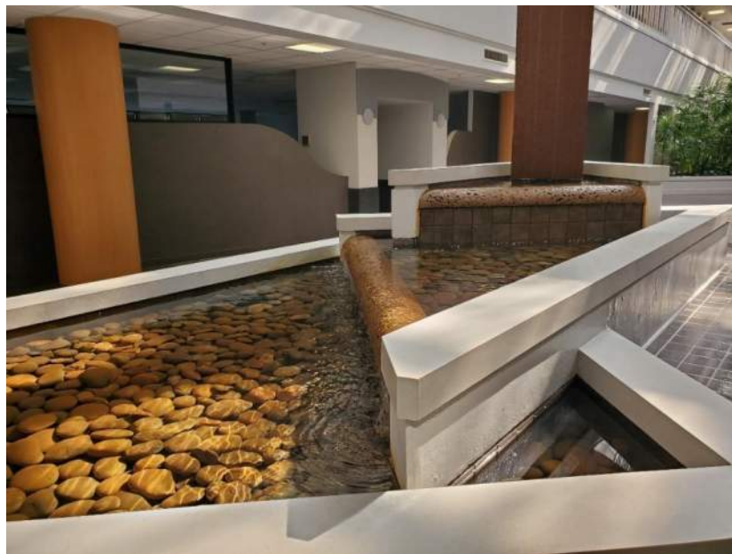
Photograph 22 – Interior flowing water unit
