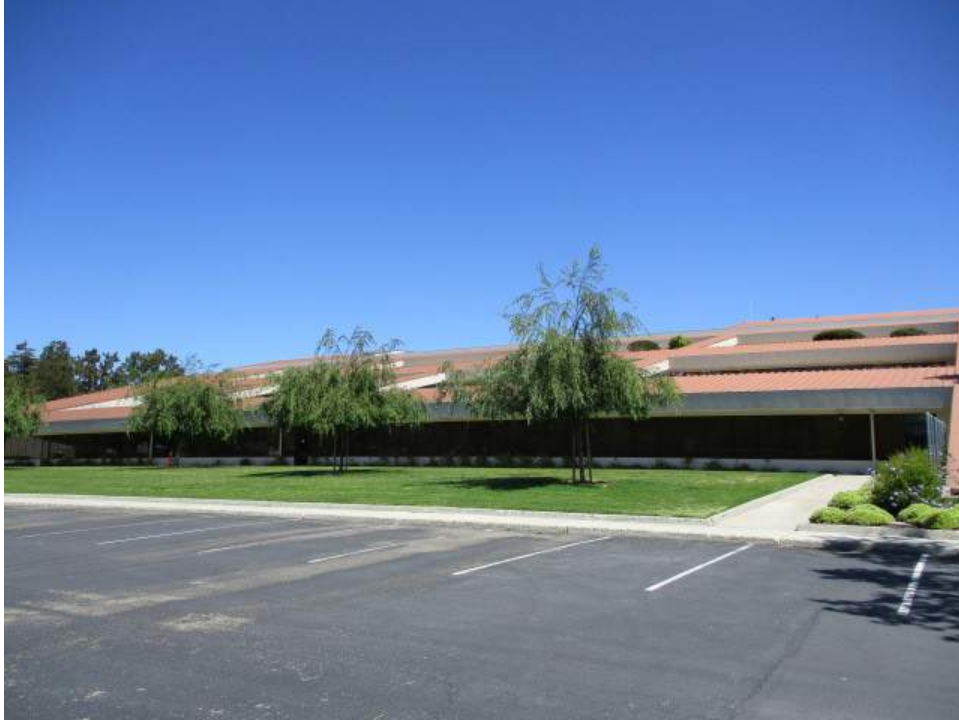
7. Southern side of the subject property building
