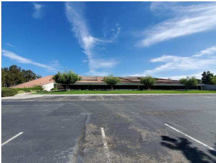
Photograph 4 – Southern side of the building, facing north from the parking lot off of Bunker Hill Lane.
