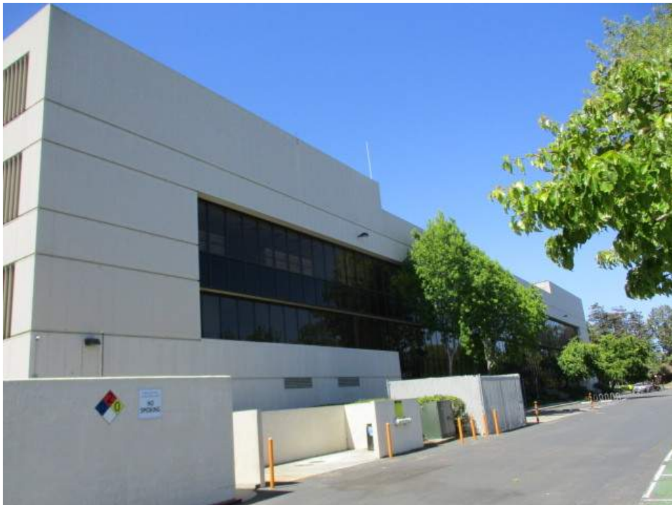
4. Northern side of the subject property building
