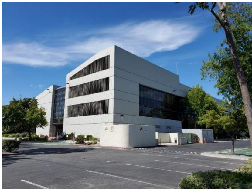
Photograph 2 – Northeastern corner of the building, facing southwest.
