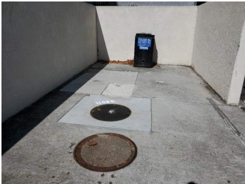
Photograph 10 – Grease interceptor and presumed former solid waste storage area on the north side of the building.
