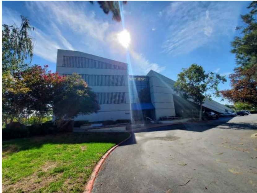
Photograph 1 – Western side of the building located at 5201 Patrick Henry Drive, facing East.
