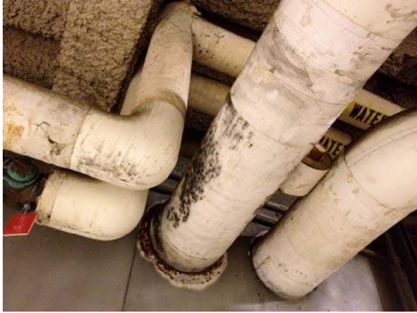
21. View of mold growth on piping within the equipment room observed April 5.
