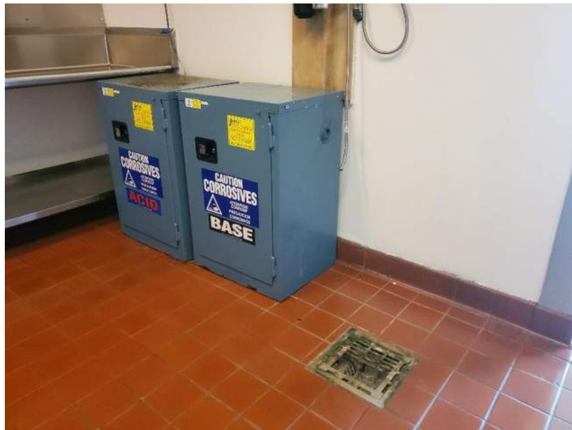
Photograph 26 – Corrosive material storage in kitchen next to floor drain
