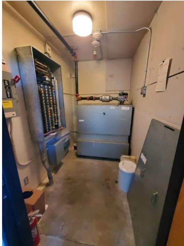
Photograph 19 – Western elevator room, facing south.
