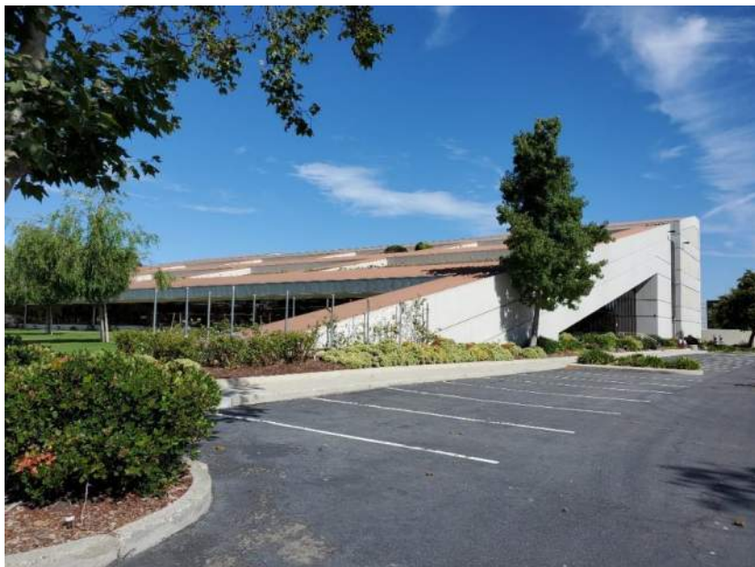
Photograph 6 – Southeastern side of the building, facing northwest from the parking lot off Betsy Ross Road.
