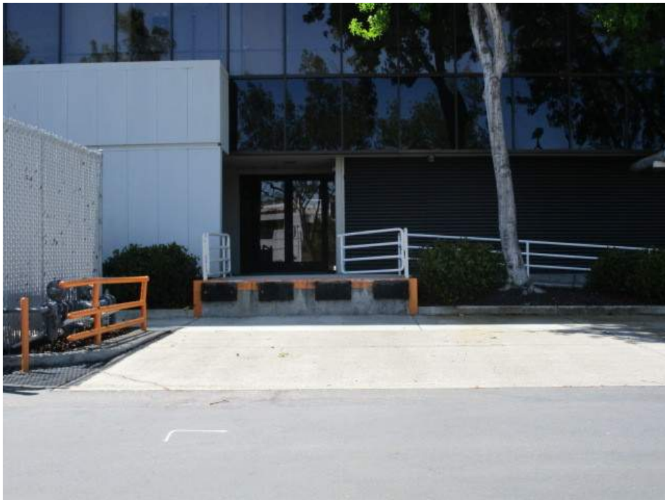
6. Loading dock on the northern side of the subject property building
