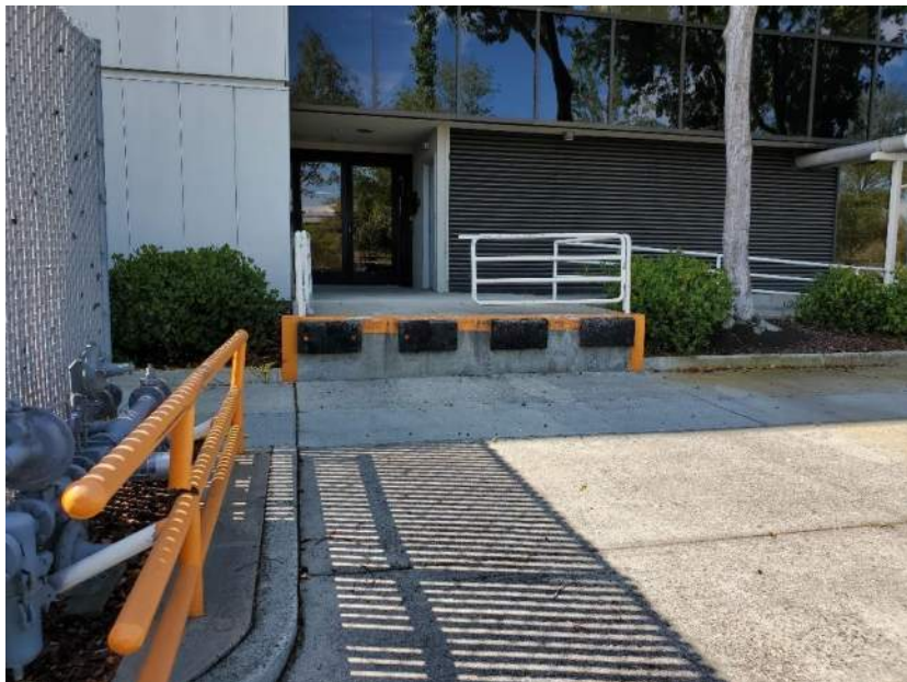
Photograph 14 – Loading dock on northern side of the building, facing south.
