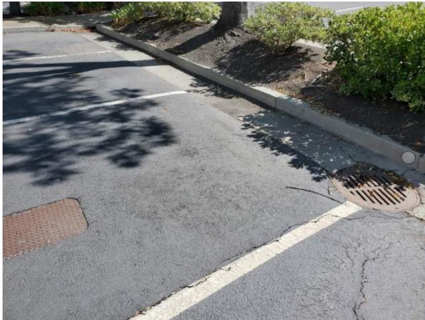
Photograph 12 – Storm drain in the asphalt parking lot.
