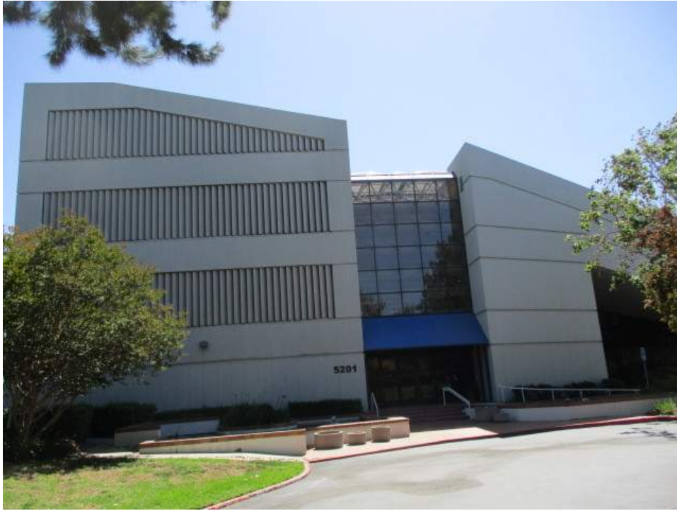
1. Western side of the subject property building
