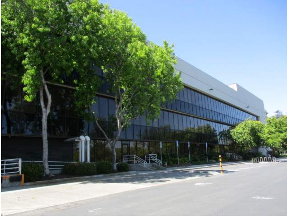
5. Northern side of the subject property building
