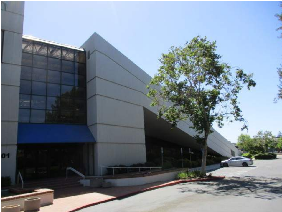
2. Western side of the subject property building
