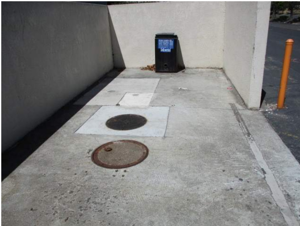
12. Current grease trap and suspect former grease trap on the northern side of the site building
