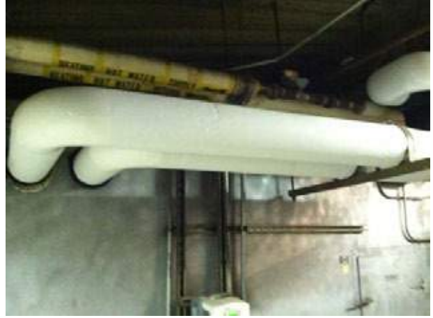
22. View of the area depicted in photograph 21 after abatement.
