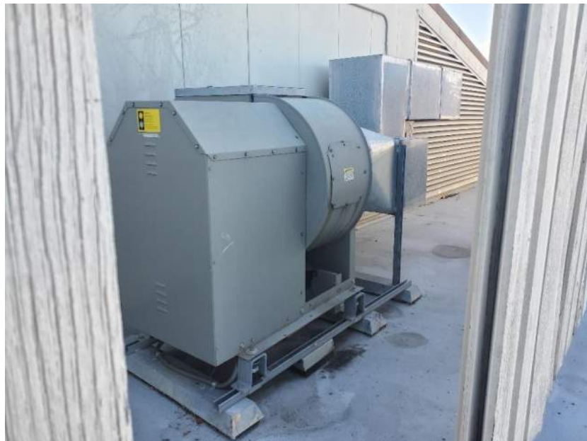
Photograph 16 – HVAC Unit on the roof, facing east.
