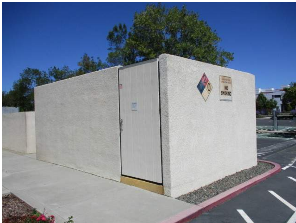
10. Enclosure with a diesel fuel-powered emergency generator northeast of the subject property building
