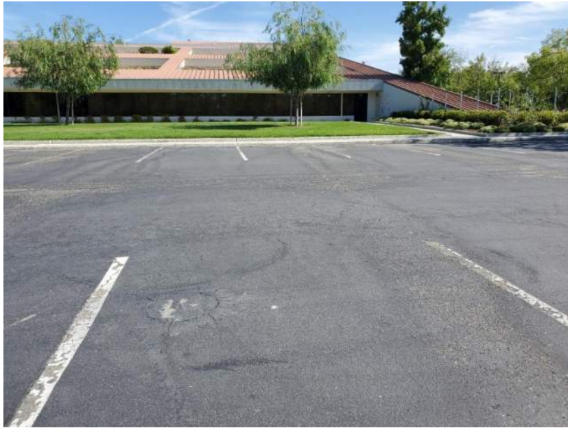
Photograph 5 – Southern side of the building, facing north from the parking lot off Bunker Hill Lane.
