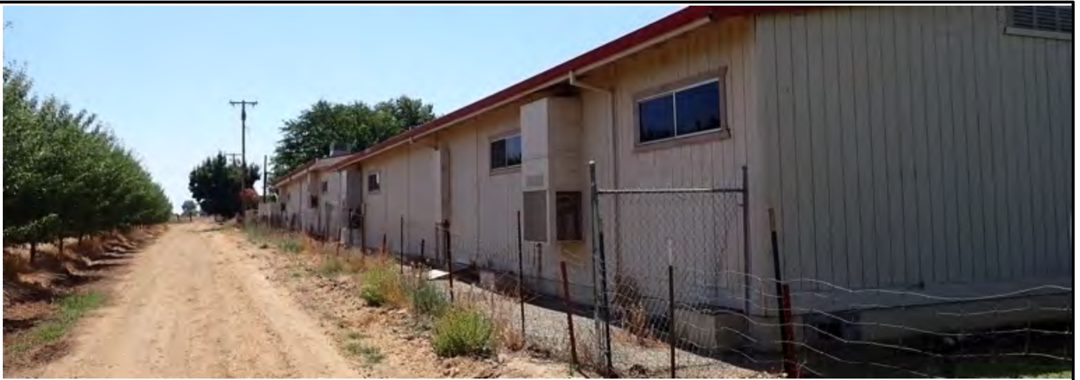
Image 4. Looking SW, four portable classrooms on the western side of subject property.
