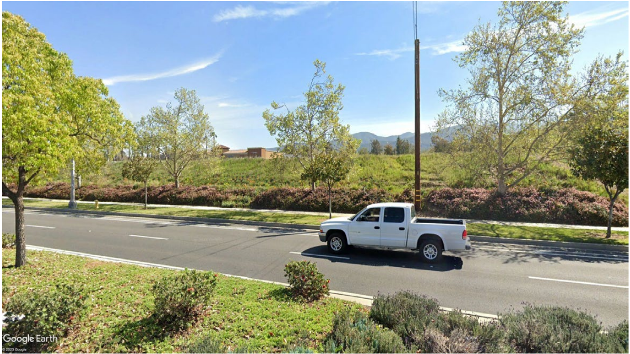
View of the northern side of project site from Foothill Pkwy.
