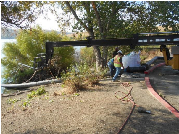
26-Making Final Connection for Discharge Pipe (10-9-20)
