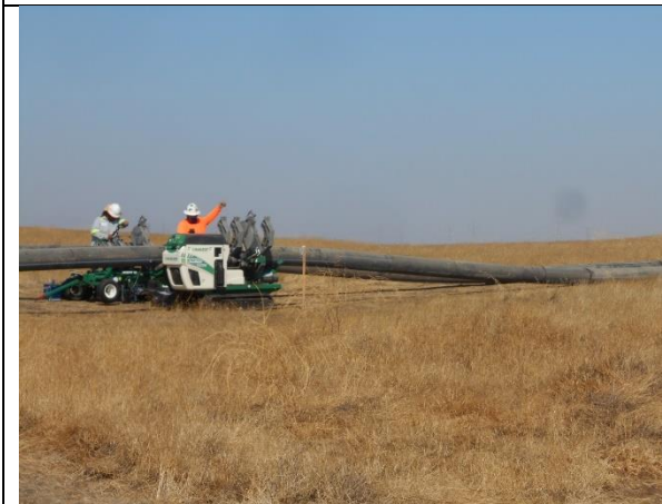
9-Completed Fusion and Moving Pipe (9-30-20)
