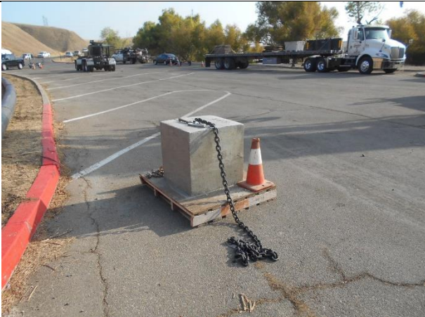
24-Concrete Anchor for Outlet (10-9-20)
