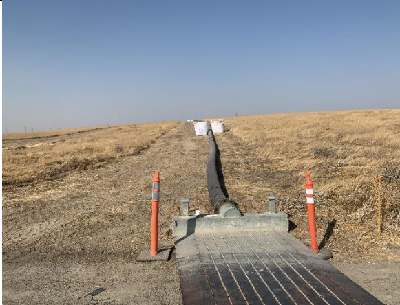
13-Pipeline before road crossing (10-29-20)
