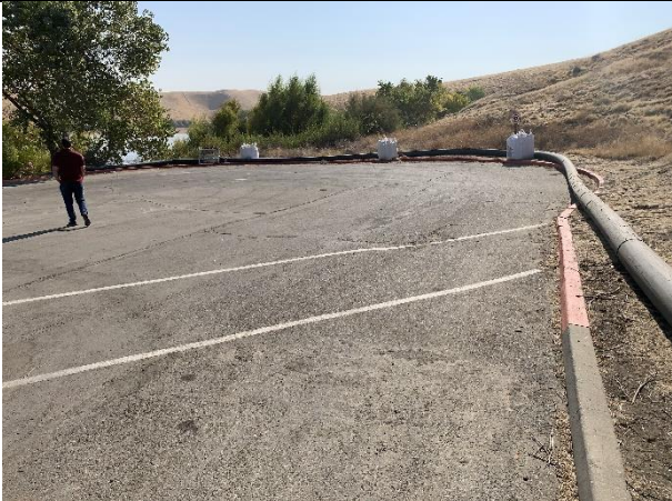
22-Pipe at end of parking area (10-29-20)
