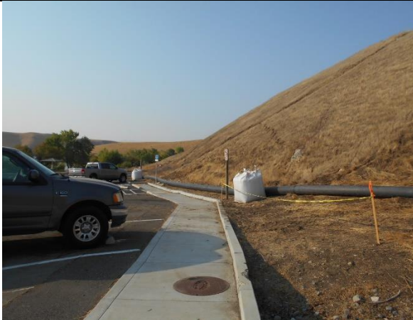
21-Sandbag Placement at Parking Lot (10-7-20)
