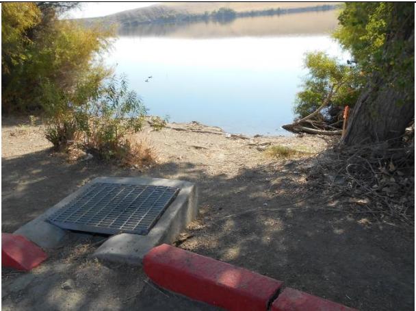
4-Outlet Location at Reservoir (9-29-20)
