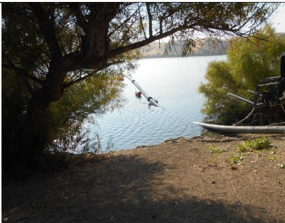
25-Moving Outlet into Reservoir (10-9-20)
