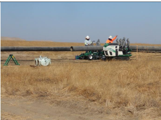
8-Removing Pipe from Fusion Machine (9-30-20)
