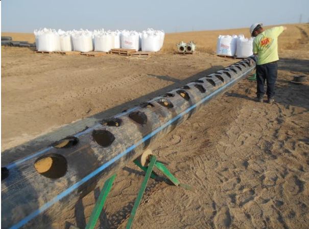
20-Outlet Diffuser Pipe Fabrication (10-7-20)
