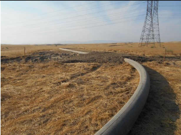
18-Ramp Over Pipe at Filters (10-6-20)
