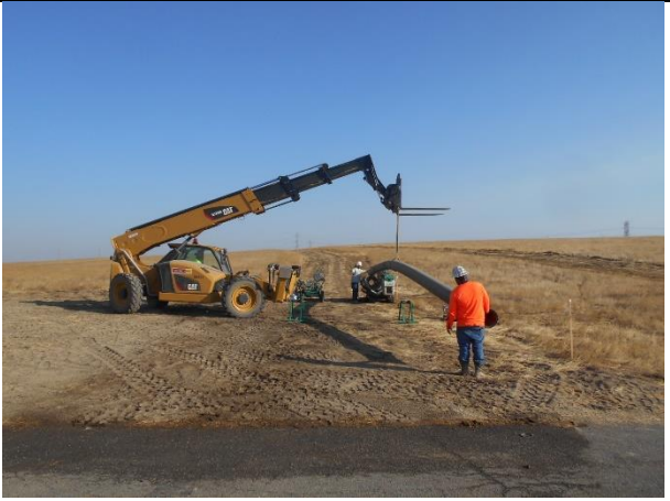
6-Placing Pipe for Fusion (9-30-20)
