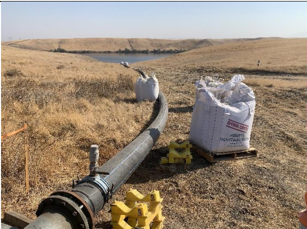
12-Pipeline after road crossing (10-29-20)
