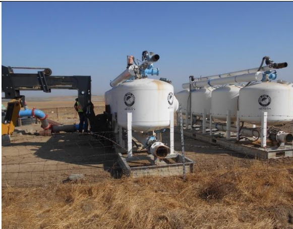
3-Filters Being Placed (9-29-20)
