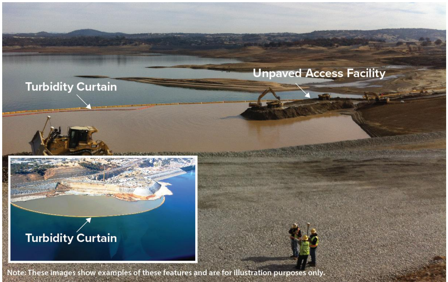
Figure 8. Examples of Turbidity Curtain and Unpaved Access Facility
