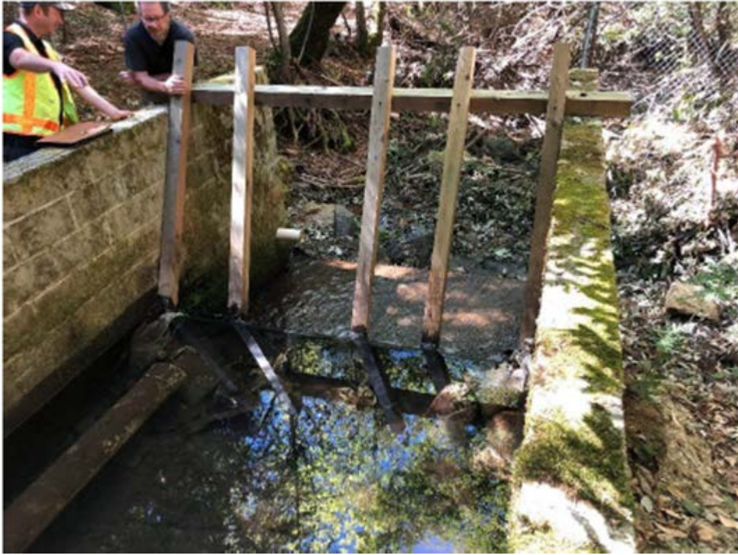
Existing Wooden Diversion Structure
