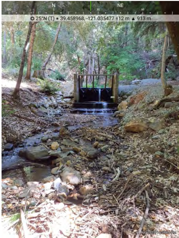
Photo 5. C-1, Looking upstream at Campbell Gulch Diversion structure.
