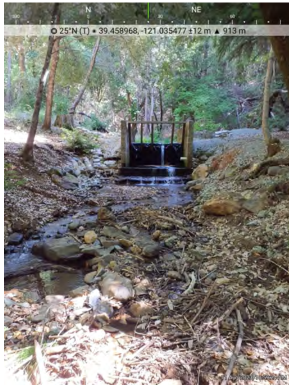
Photo 3. C-1, Looking upstream at Campbell Gulch Diversion structure.
