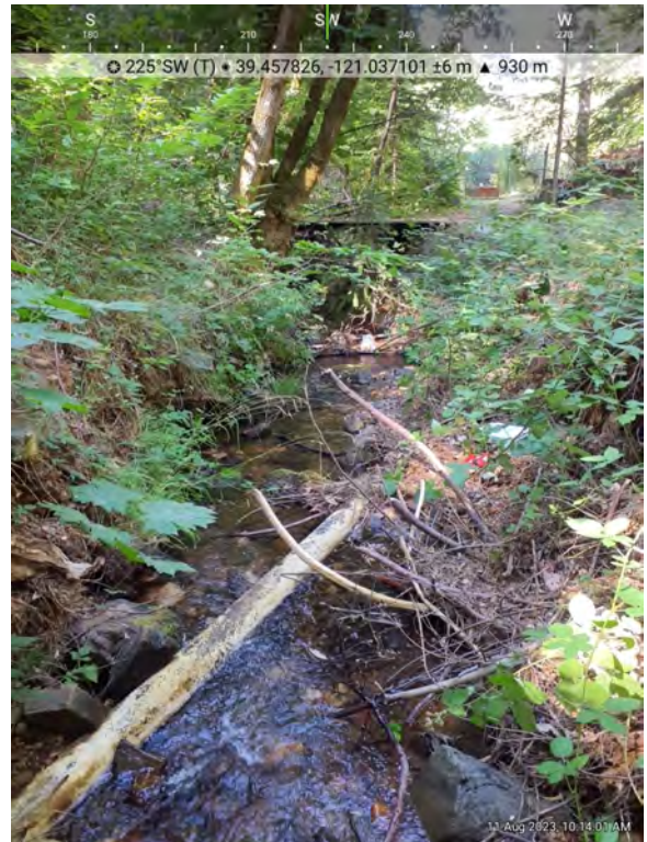
Photo 4. C-2, Looking downstream at Campbell Gulch pipe location.
