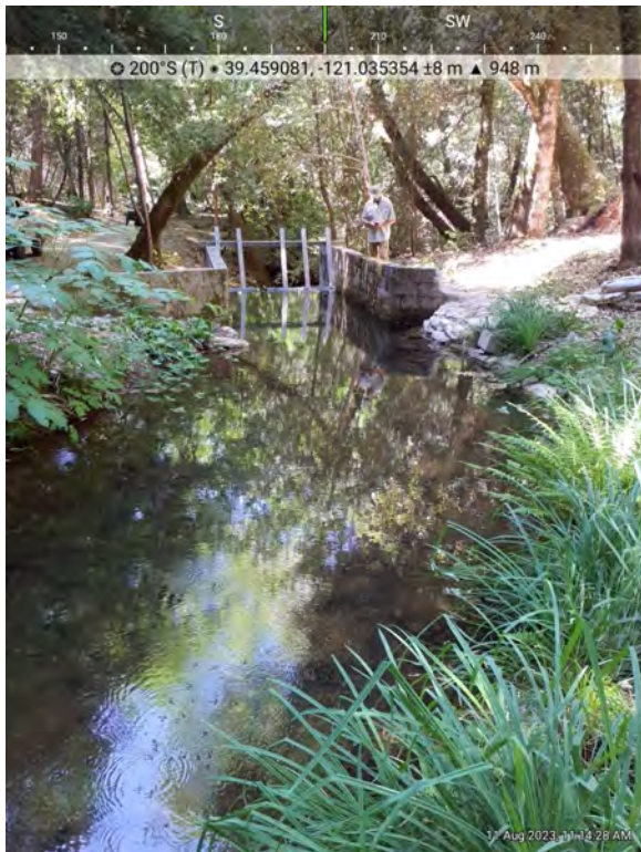
Photo 7. C-1, Looking downstream at Campbell Gulch Diversion structure.
