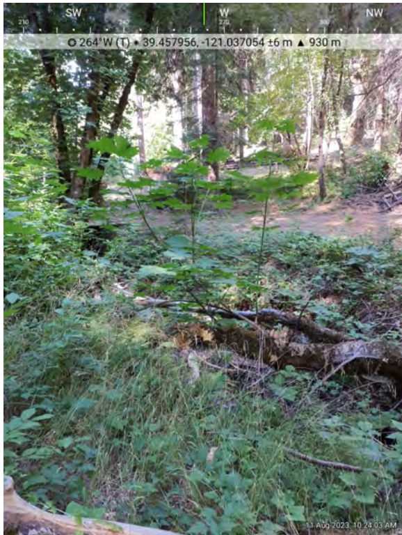
Photo 3. C-2, Looking across Campbell Gulch along pipe excavation alignment.
