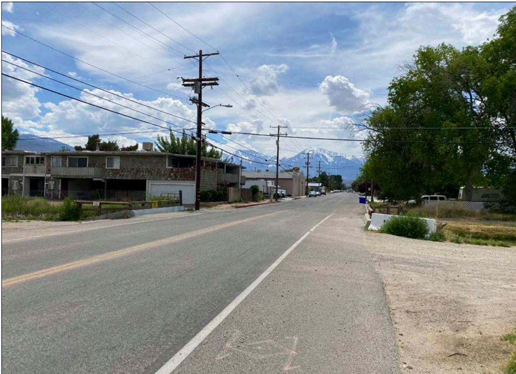
Photo 8. View looking west toward the bridge on East Line Street.
