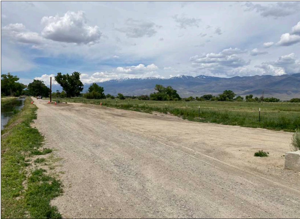
Photo 5. View of the unpaved access road along the canal north of East Line Street.
