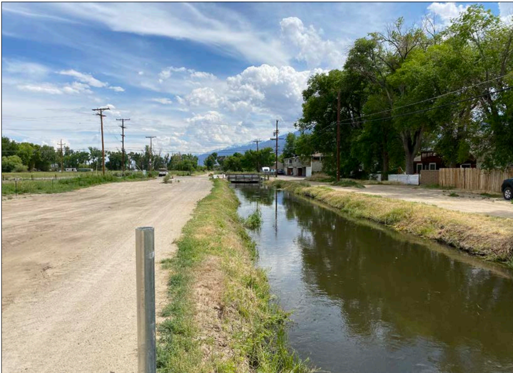
Photo 6. View of the Bishop Creek Canal looking south towards the East Line Street Bridge.
