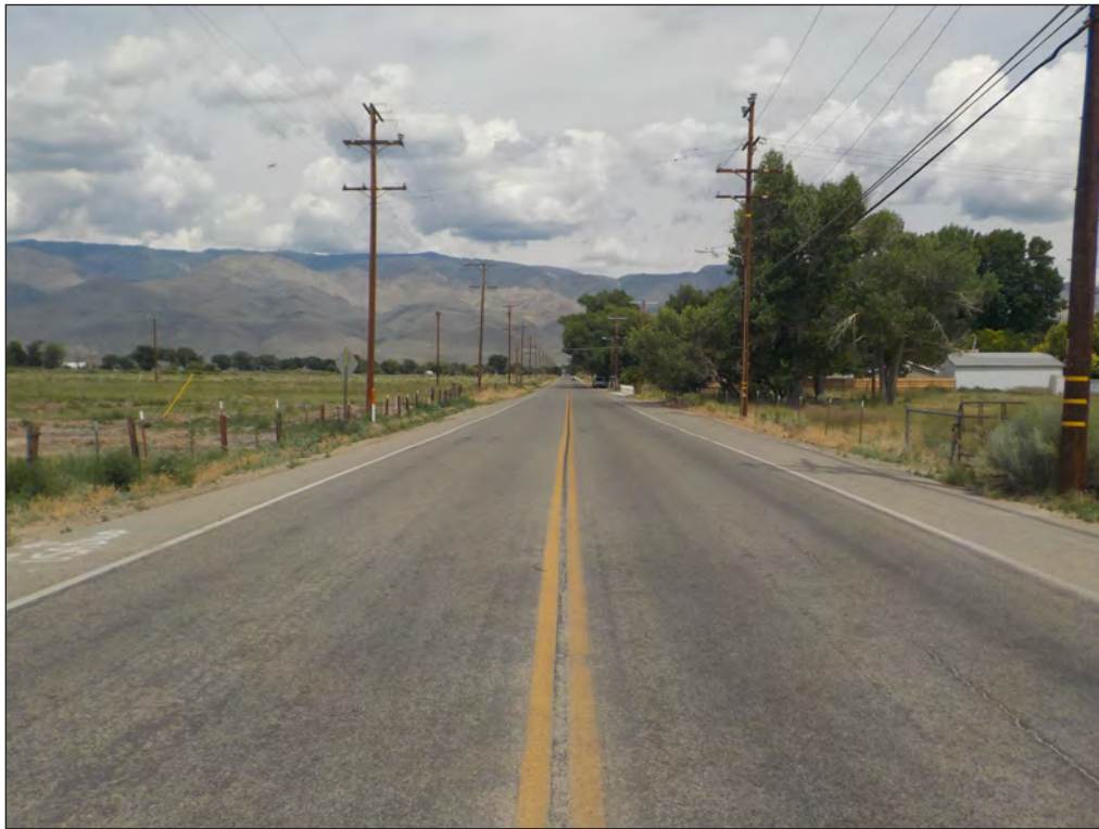
Photograph 3. Overview from center of East Line Street facing East, taken on June 15, 2023 – facing East.
