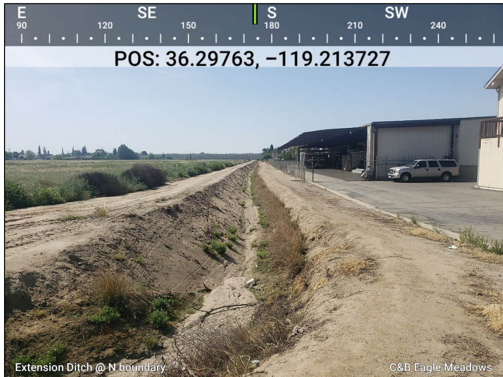
Figure 3. Overview along the northern boundary of the Project APE, looking south..
