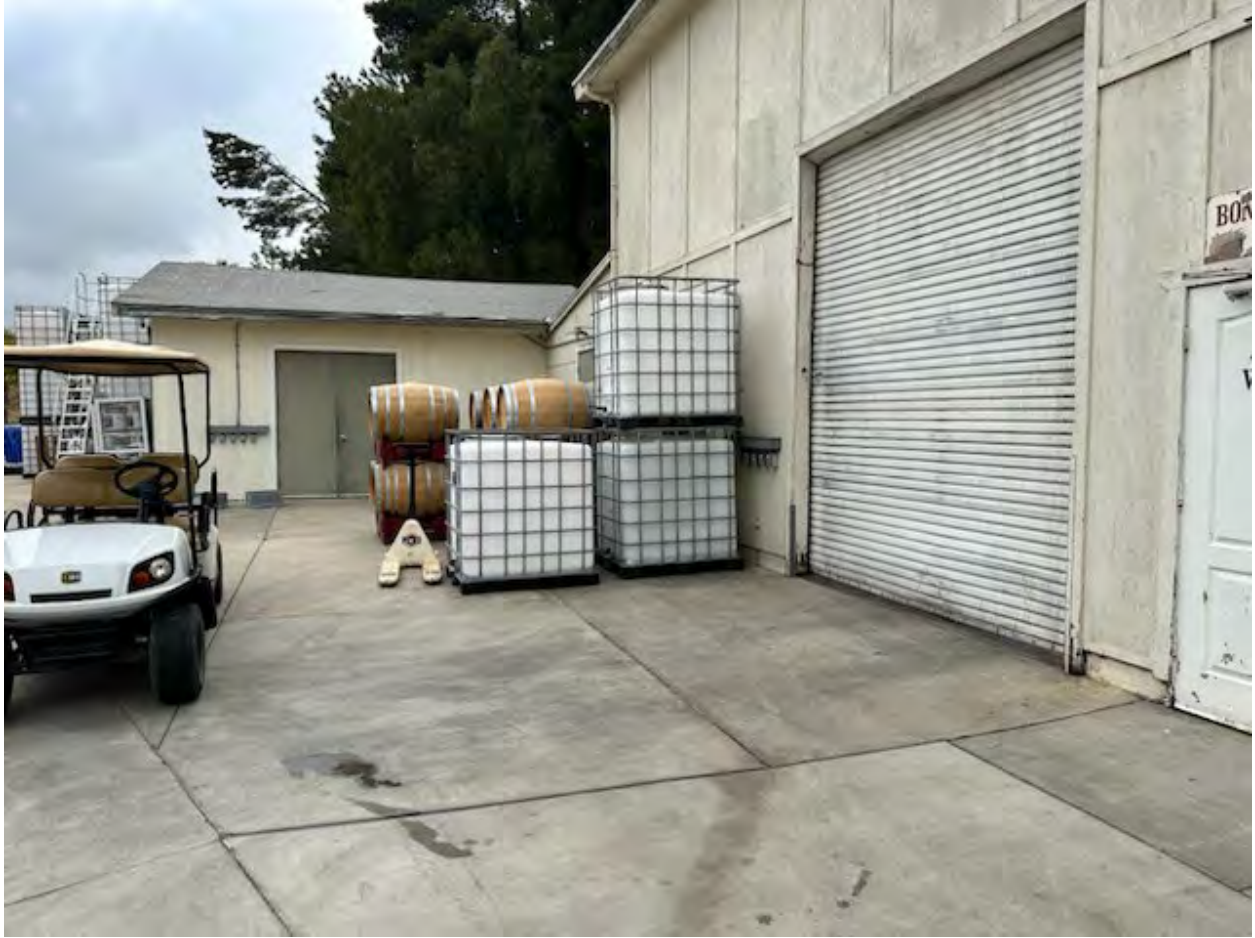
Exterior of Wine Production Building.
