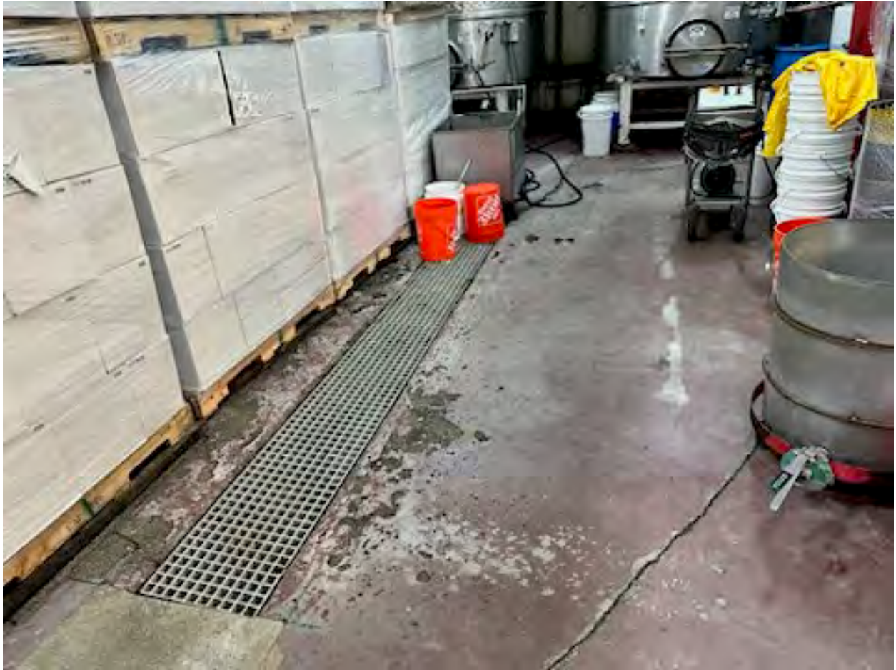
Interior drain of Wine Production Building.
