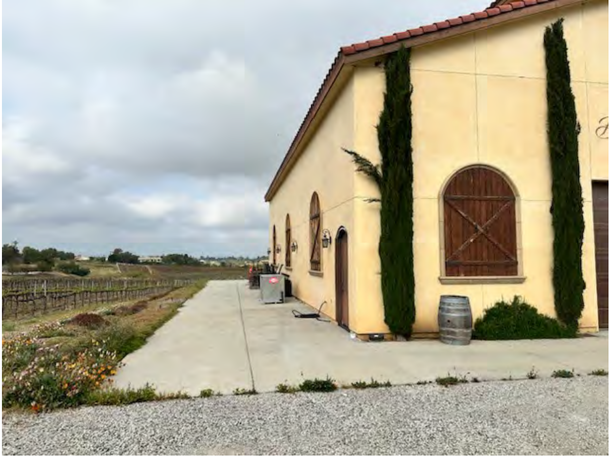
Southern portion of Barrel Room, looking west.
