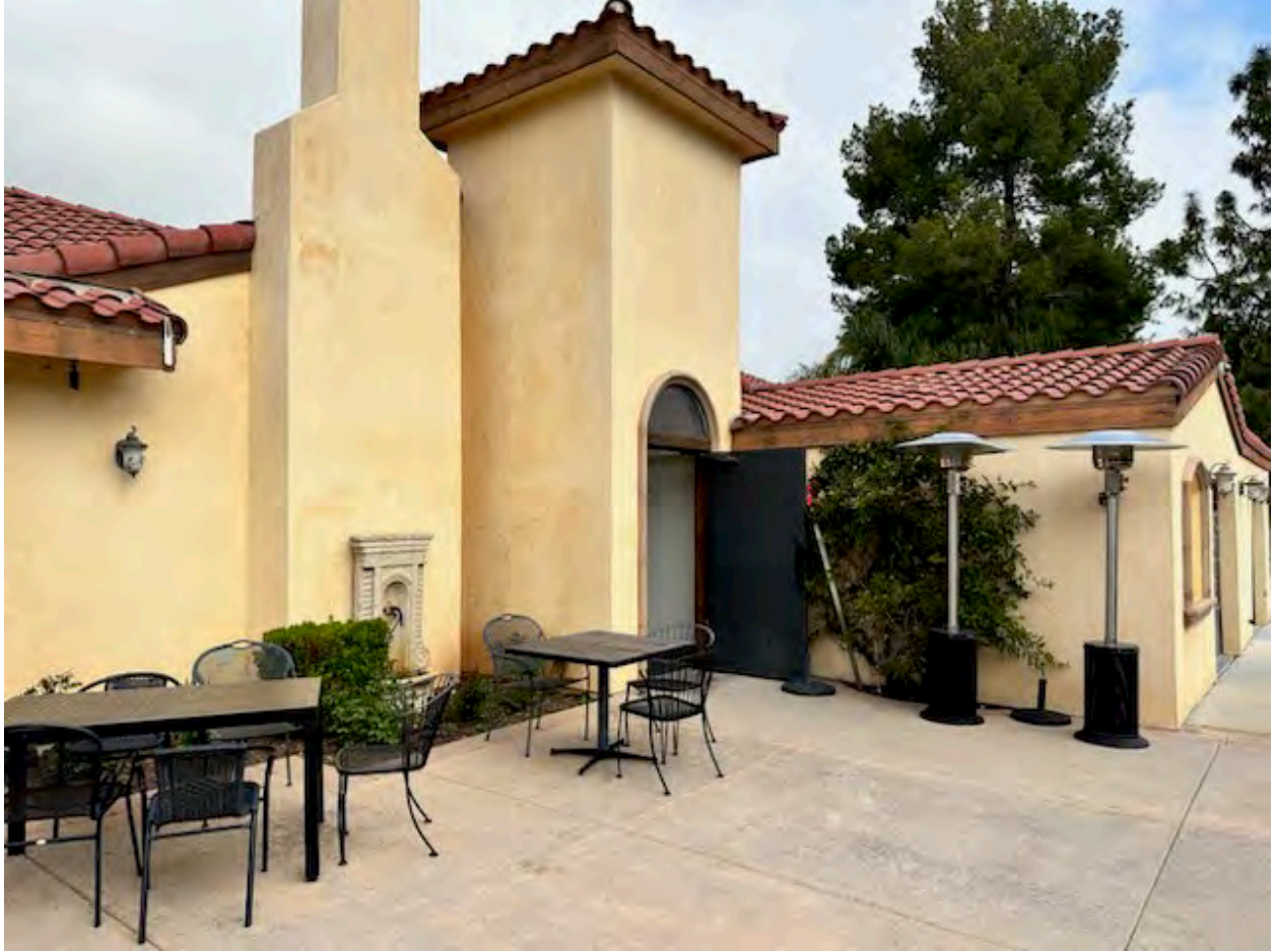
Former single family residence converted into the Clubhouse, located southwest of the Wine Tasting Room.
