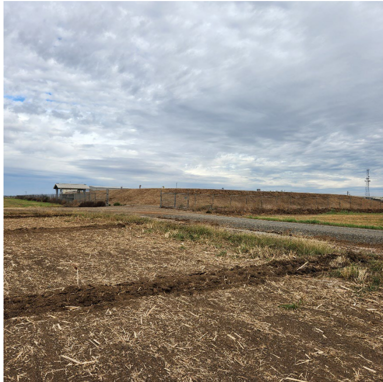
Photo No. 15 View to the northeast of northern extent of site; off-site adjoining property wastewater treatment plant
